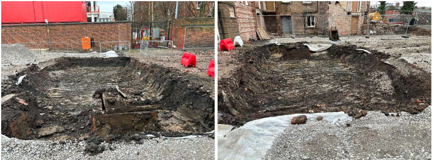
Location WS04 Excavated
