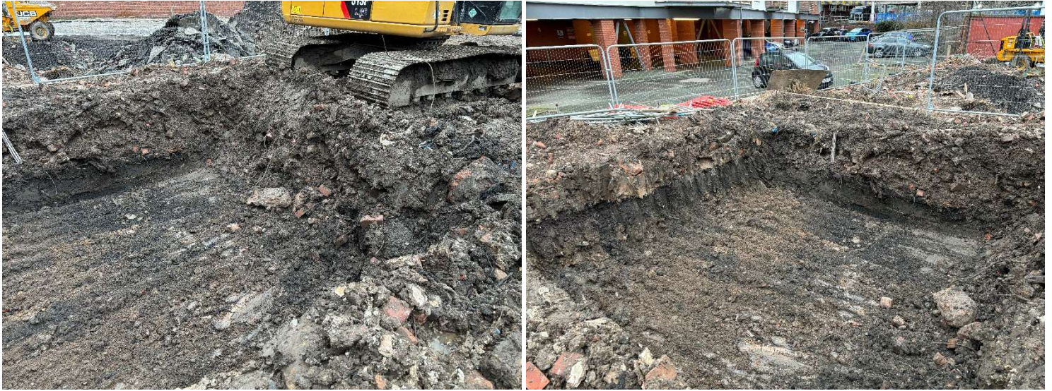
Location WS02 Excavated
