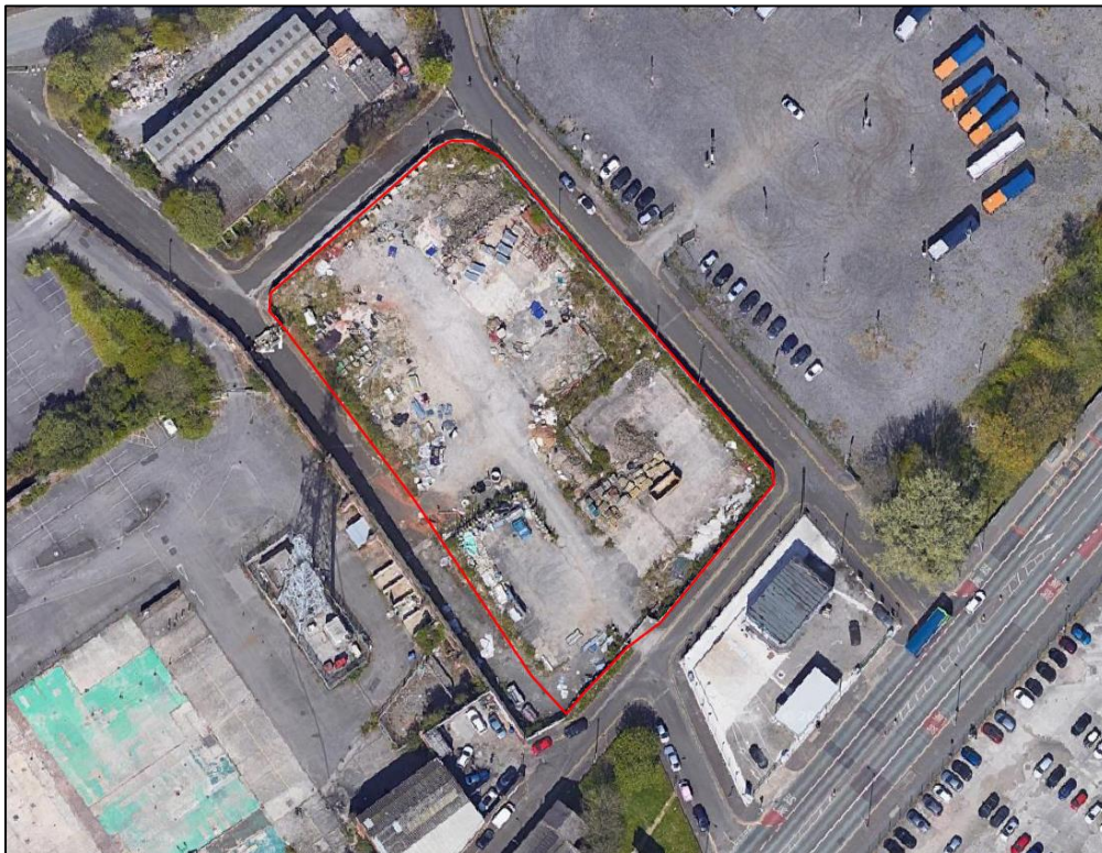
Figure 1.1 - Site red line boundary (Aerial imagery © google 2023).
