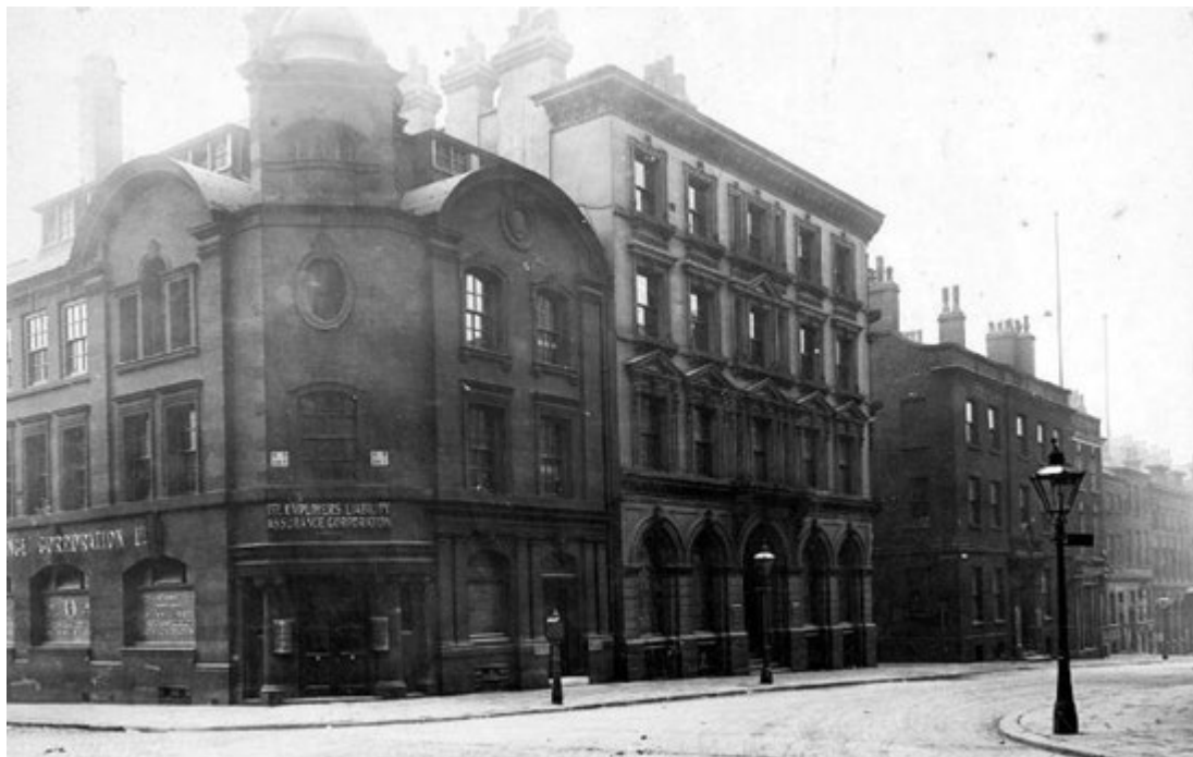
Figure 4: Site of 100 King Street in 1924 showing the earlier building upon the street. (Source: Manchester Archives)
