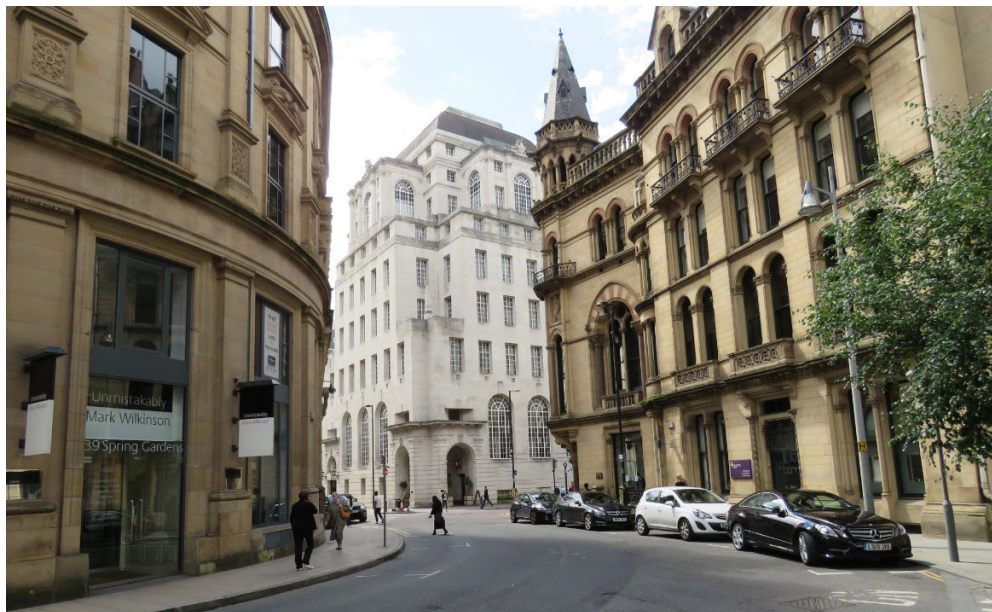
Figure 12: View of 100 King Street illustrating the prominence of the building from surrounding streets. (Source: SLHA)
