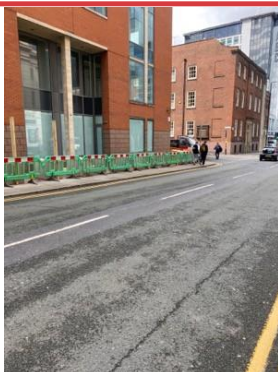
ISSUE 2 Highway photograph showing existing cracking to tarmac and temporary barriers installed on footpath in preparation for hoarding erection - Quay Street looking towards Byrom Street.
