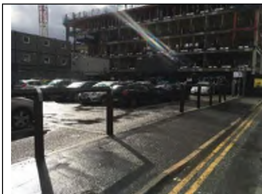
Photograph 1: View of site and site access from Cross Keys Street,
