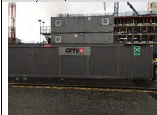
Photograph 3: Temporary site cabins located in eastern area of site.
