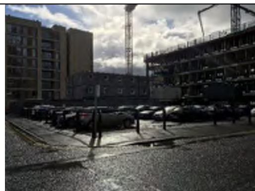
Photograph 2: View of site from north western corner.
