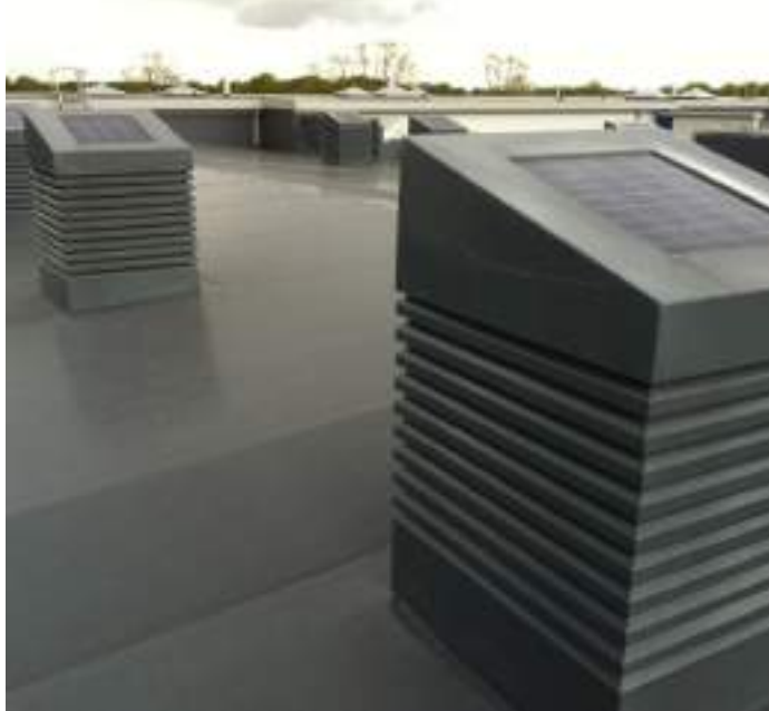
Windcatcher roof vents
