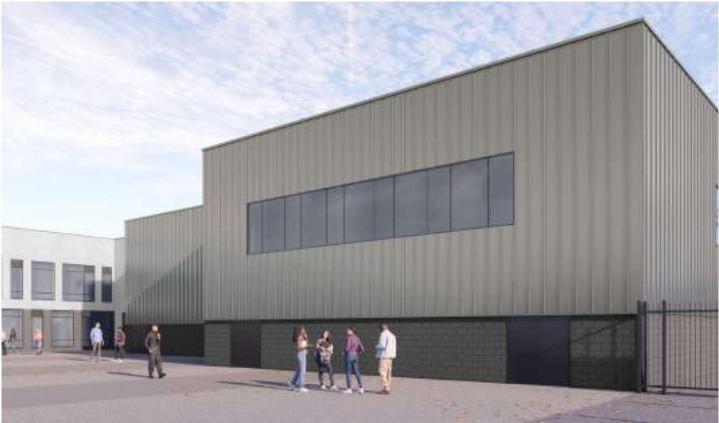
View onto Sports Hall North East Elevation - Standing Seam Cladding
