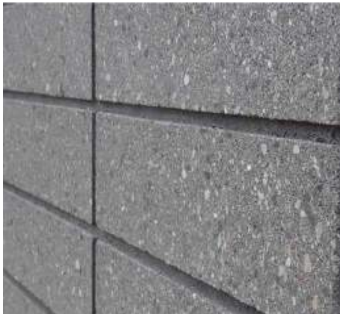
Shot blasted concrete blockwork
