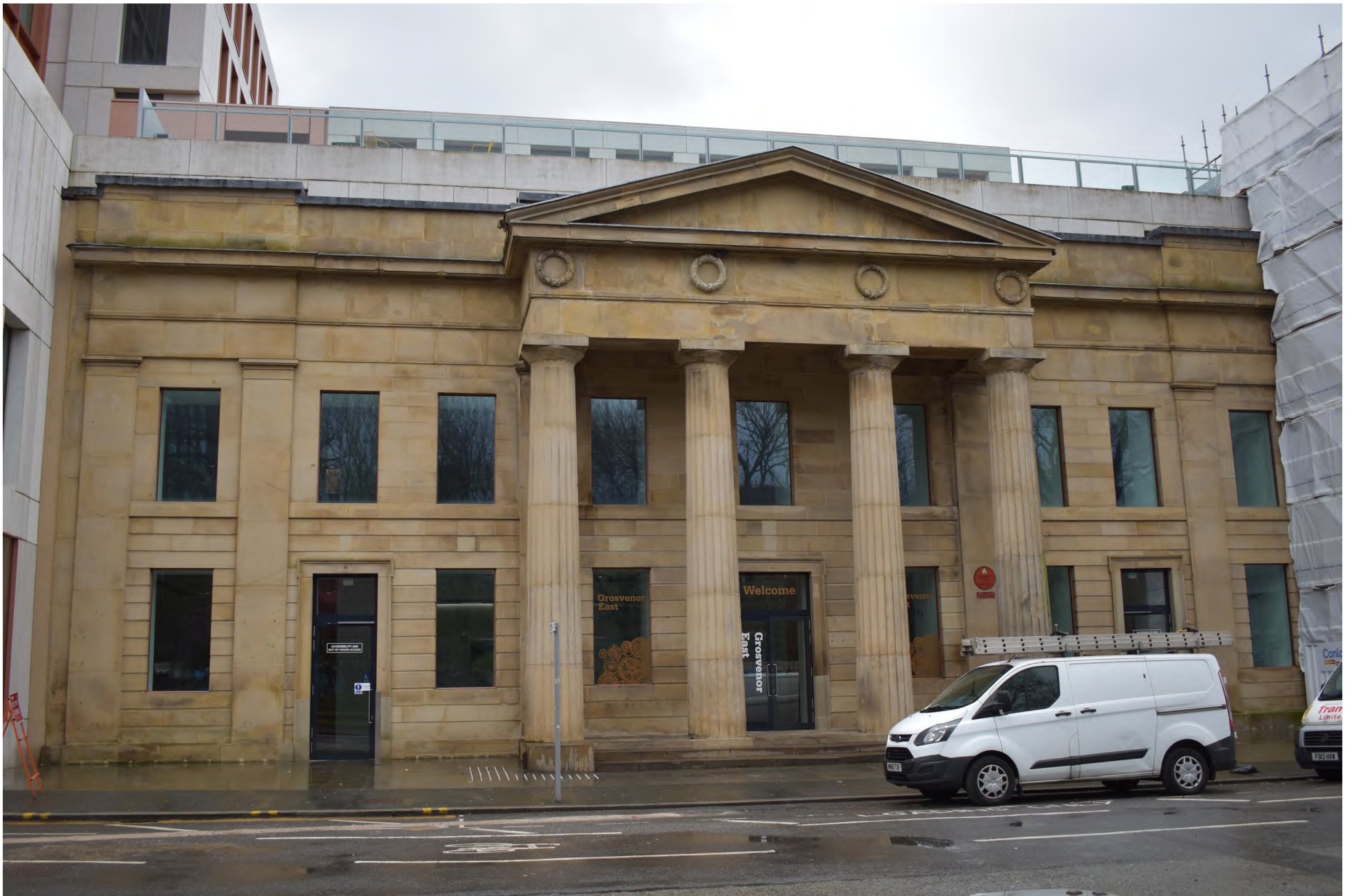
5. Former Town Hall facade (Grade II)
