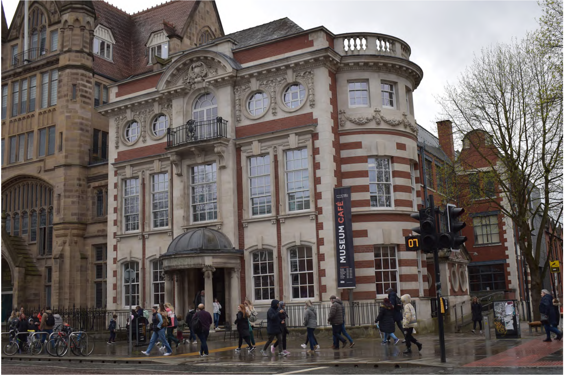
9(b). Former Department of Metallurgy (Grade II)
