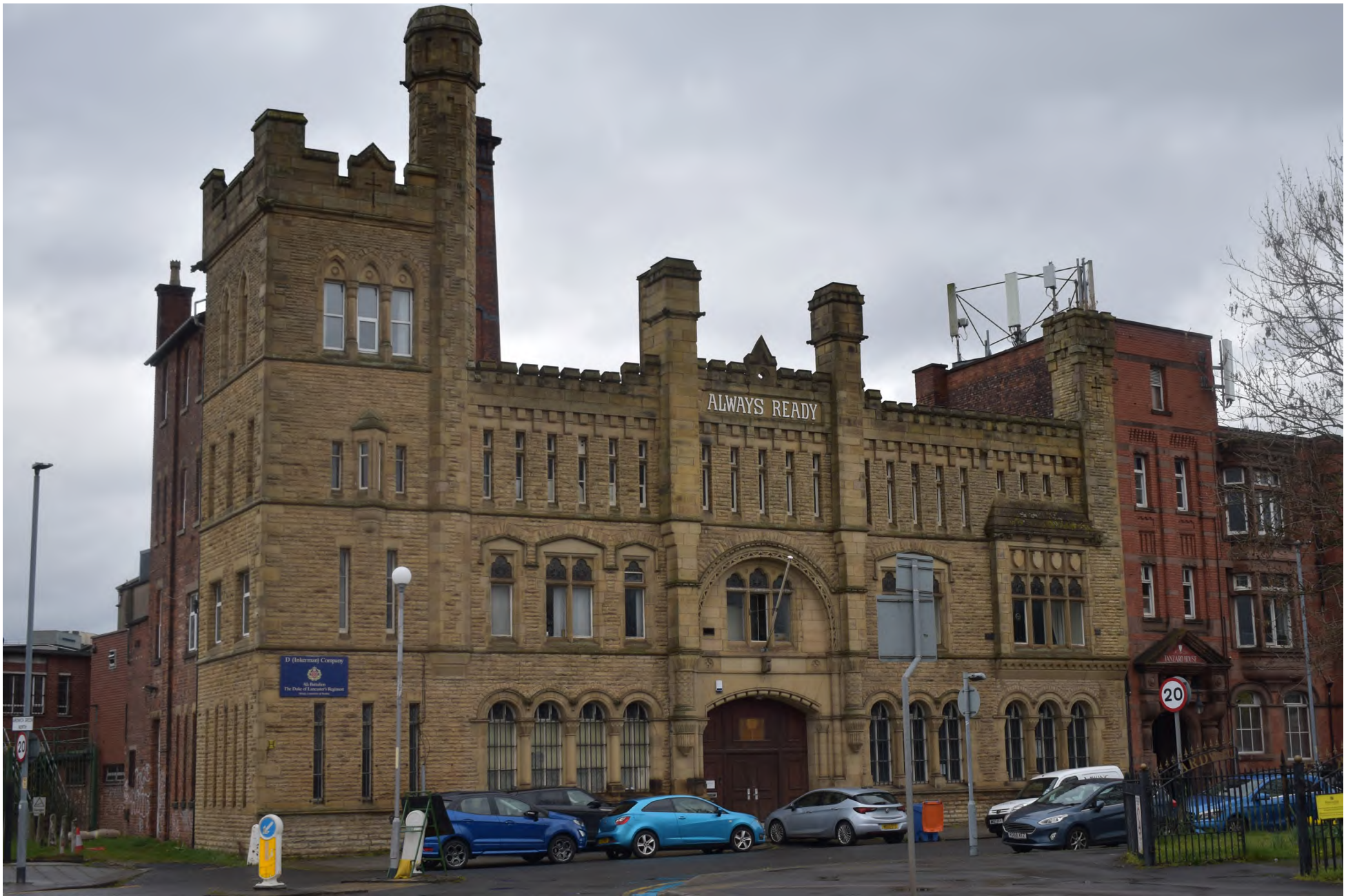
20. Drill Hall (Grade II)
