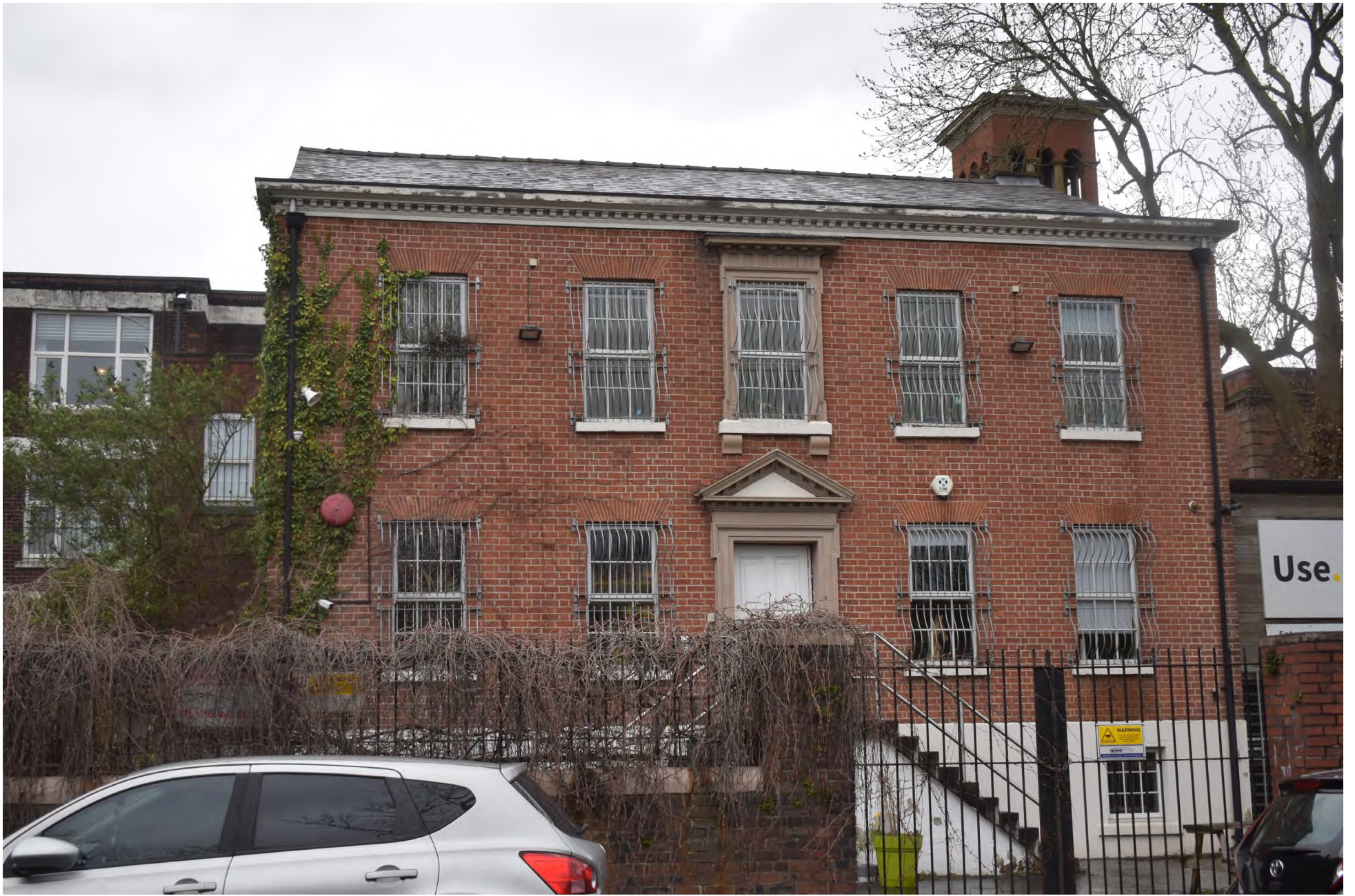
24. No.31 Ardwick Green North (Grade II)
