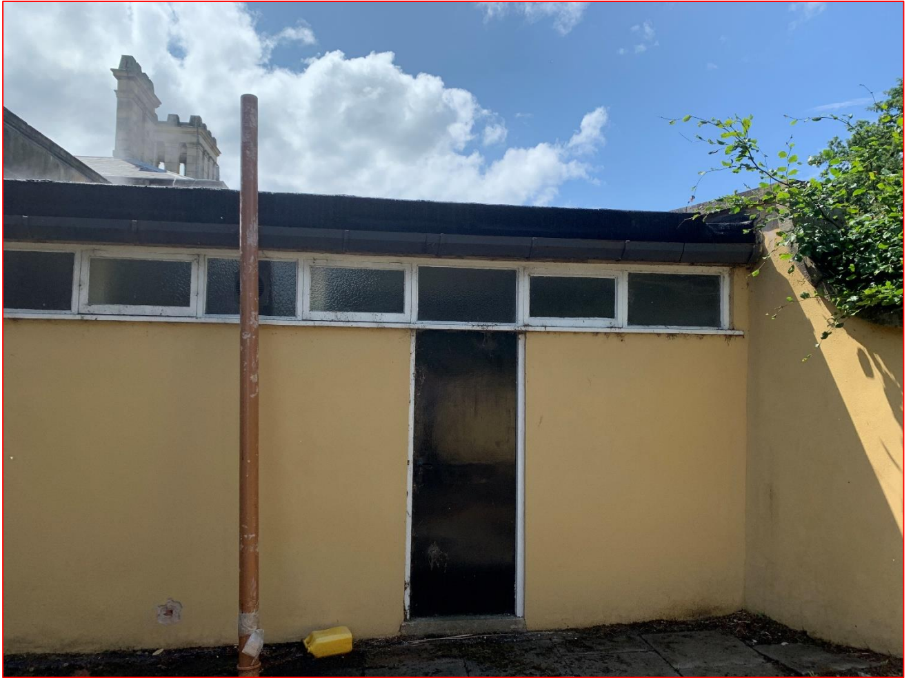
Plate 8 – Part view of the late 20 th century toilet block, which is attached to the north elevation of the Orangery. Note that this view shows the east elevation to the toilet block.
