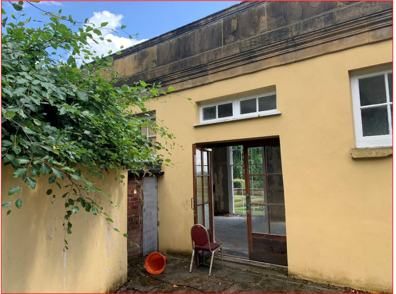
Plate 7 – Part view of the north elevation to the Orangery. Note that this view is taken from within the enclosed courtyard area.
