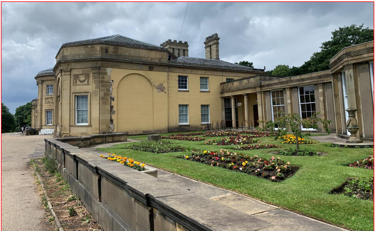
Plate 3 – Part view of the east elevation to Heaton Hall. Note that the western part of the south elevation to the single-storey Orangery is evident in centre-right of picture.
