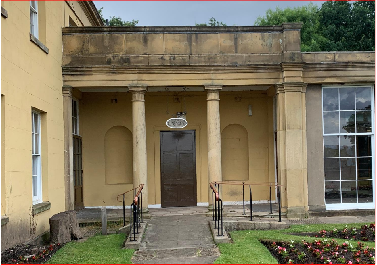
Plate 6 – View of the westernmost pavilion with colonnaded loggia to the south elevation of the Orangery.
