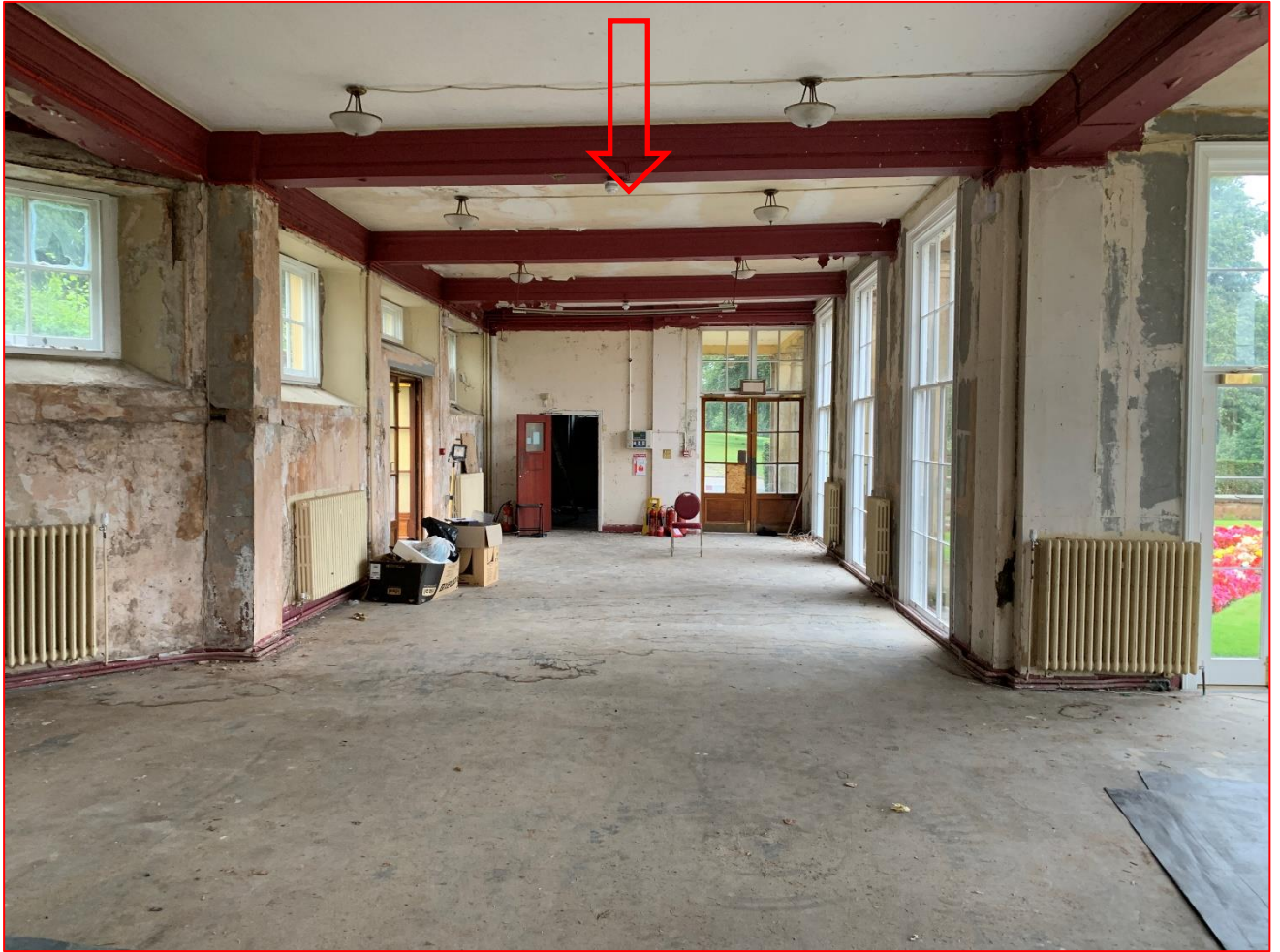
Plate 11 – View of the main interior space to the Orangery. Note that this picture is taken from the central bay looking east (towards eastern end of the Orangery). Note that the pier that supported the original dome (both removed) and associated partitioning would have been located to the left and right of the arrow.
