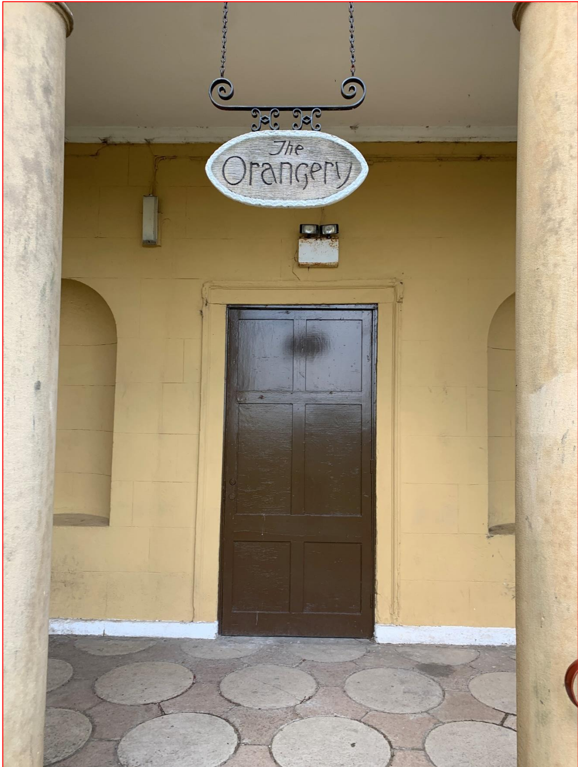
Plate 9 – View of existing door to the western pavilion of the Orangery.
