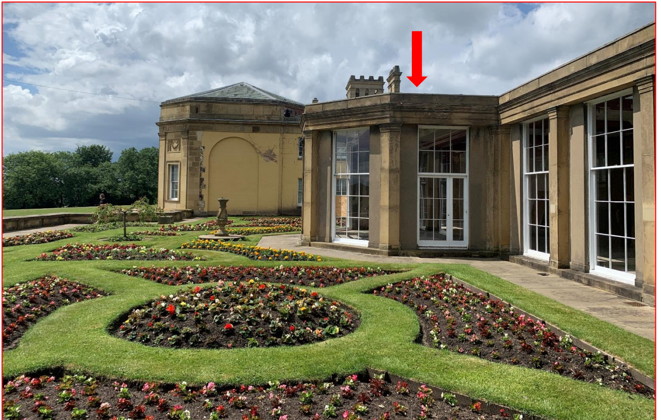
Plate 5 – View of the east side of the central bay (arrow) to the south elevation of the Orangery. Note that this view is taken looking west.
