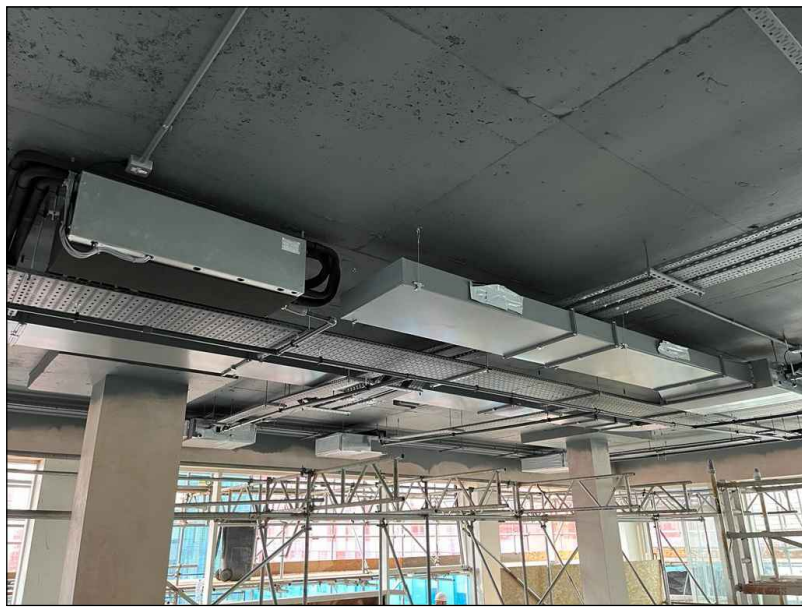
WORKMANSHIP EXAMPLE OF NEAT EXPOSED VENTILATION INSTALLATION USING DUCTWORK HANGERS CONTRACTOR TO ACHIEVE SIMILAR FINISH
