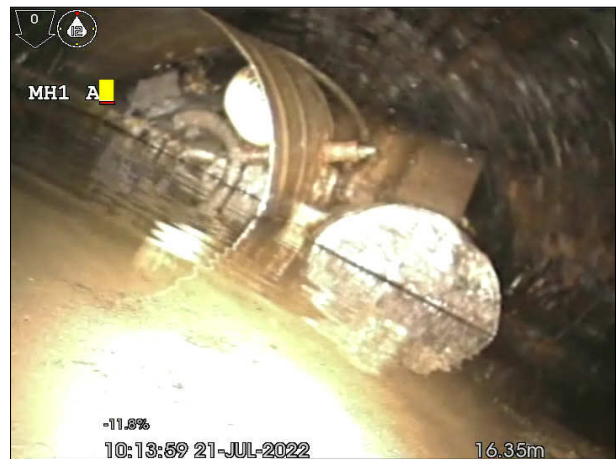
Photo: 13_13a, 00:00:00 18m, General Observation, Remark: Obstruction.
