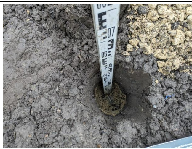
Hand dug pit HP2: Internal view of excavation
