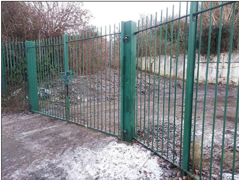
P6: Photograph showing access gate and retaining wall structure in northern part of the site.
