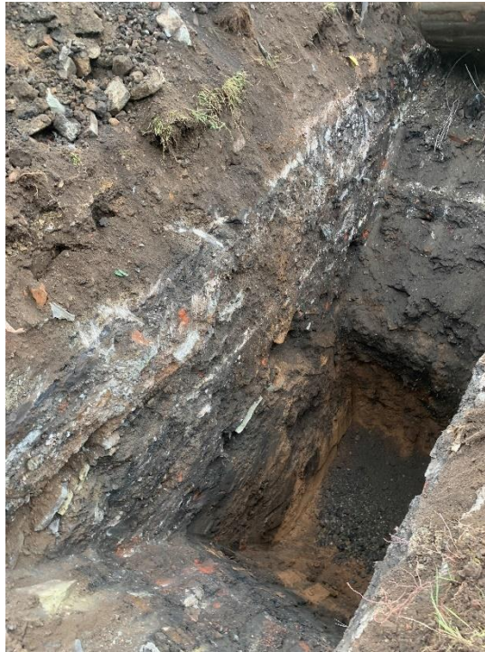
PLATE 5 EXCAVATION FOR CULVERT TRENCH (EASTERN SECTOR)
