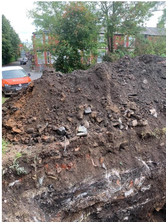
PLATE 4 EXCAVATION FOR CULVERT TRENCH (EASTERN SECTOR)
