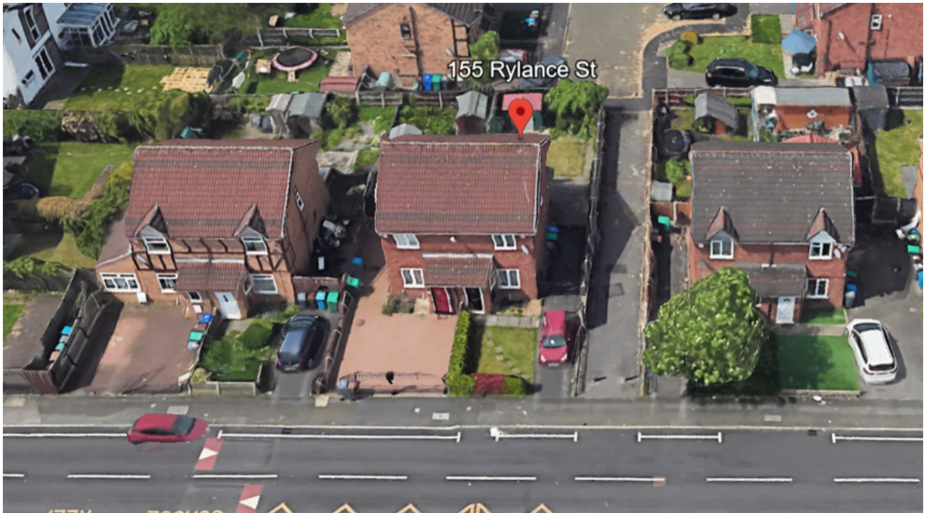
Figure 9. Extract from Google Earth, depicting the appearance of the application property in relation to the adjoining semi and the public alleyway.
