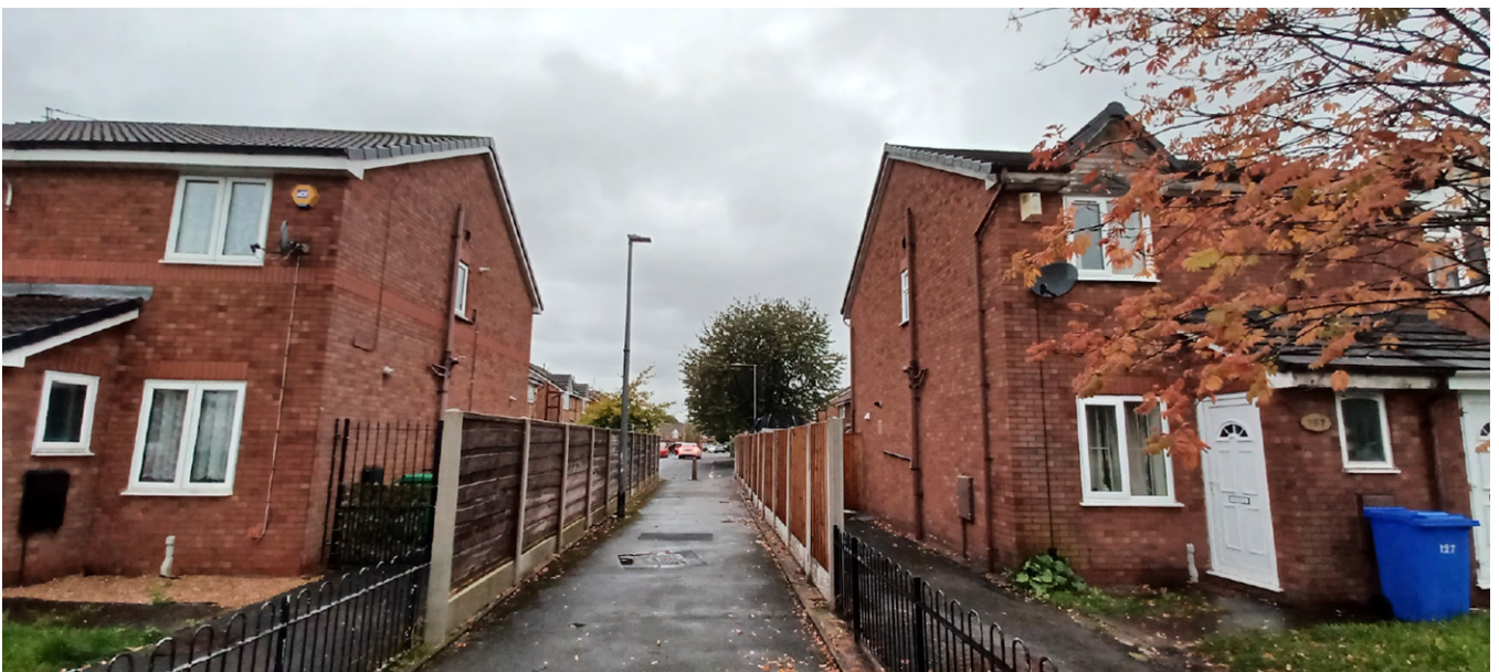
Figure 4. View along side of property and public alleyway.
