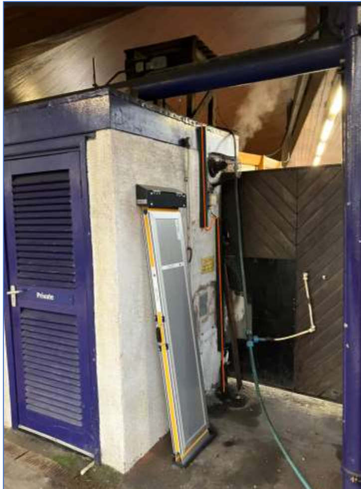
Figure 6 - Existing cable route down side of boiler room (route shown in red)
