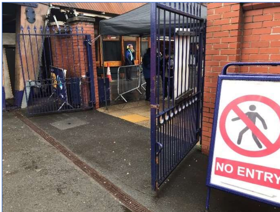
Figure 7 - View of cable chamber and cable containment fixed to rear face of canopy support column
