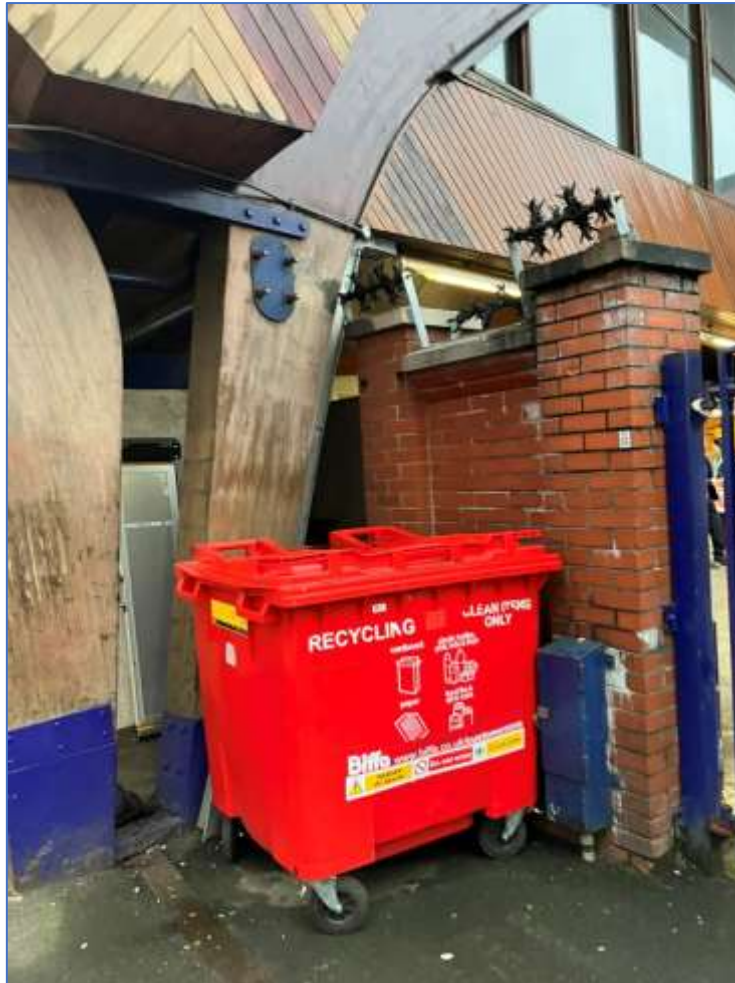
Figure 8 - Cable containment fixed to rear face of canopy support column
