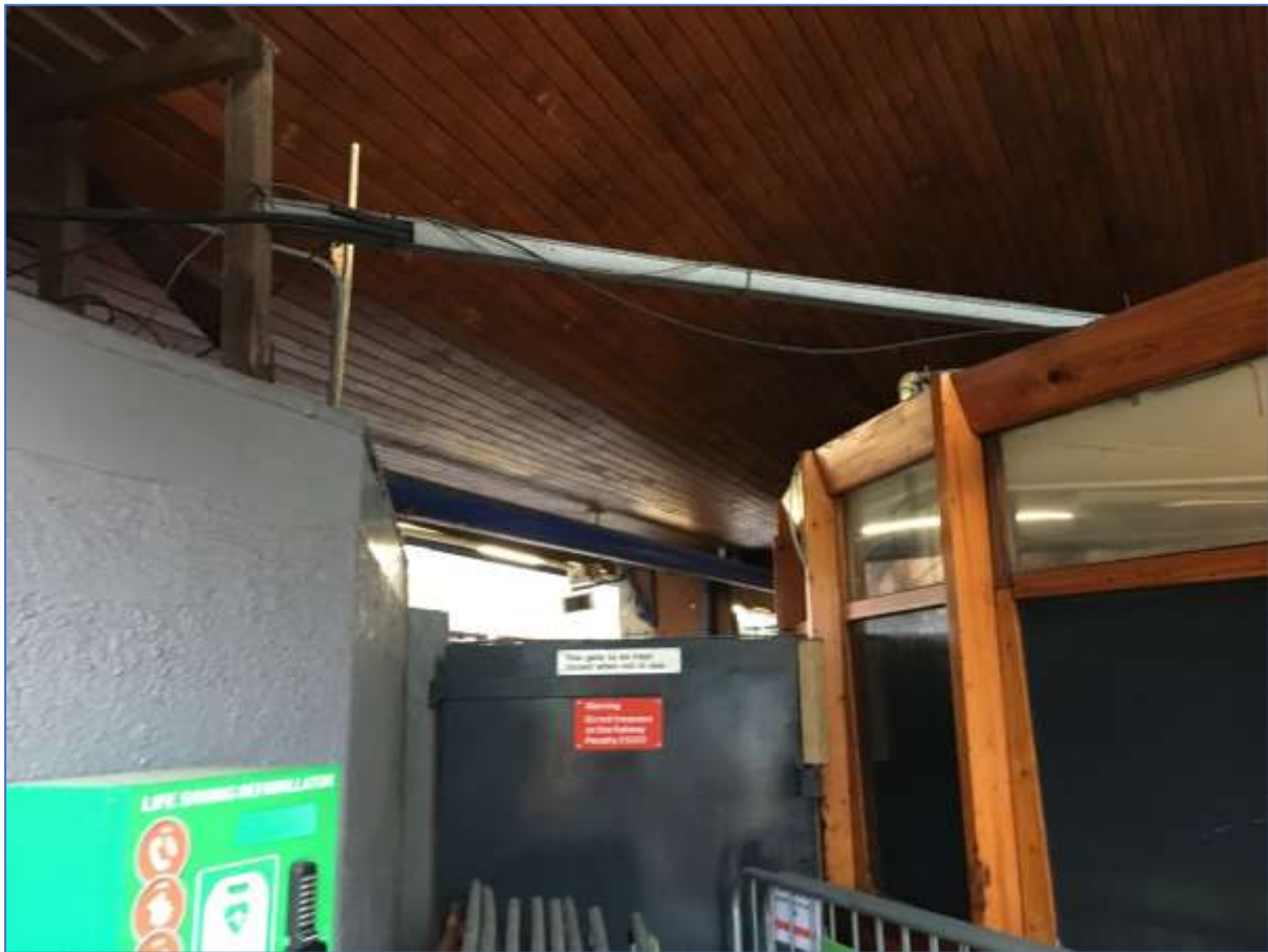
Figure 5 - Existing cable containment (boiler room on left and ticket office on right)
