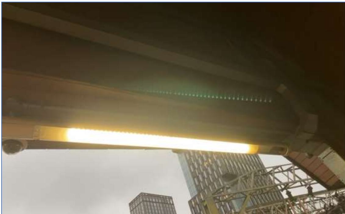
Figure 9 - View from ground level of cable containment on rear face of canopy support member meeting galvanized steel conduit for CCTV camera on underside of canopy
