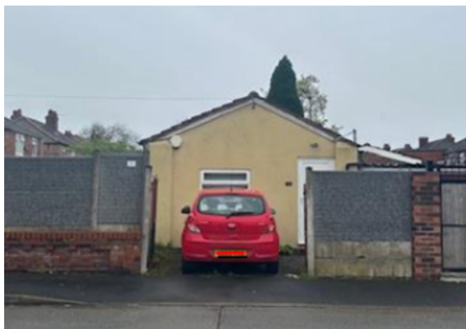
Figure 1: The application property, No. 11 Rose Cottage Road.
