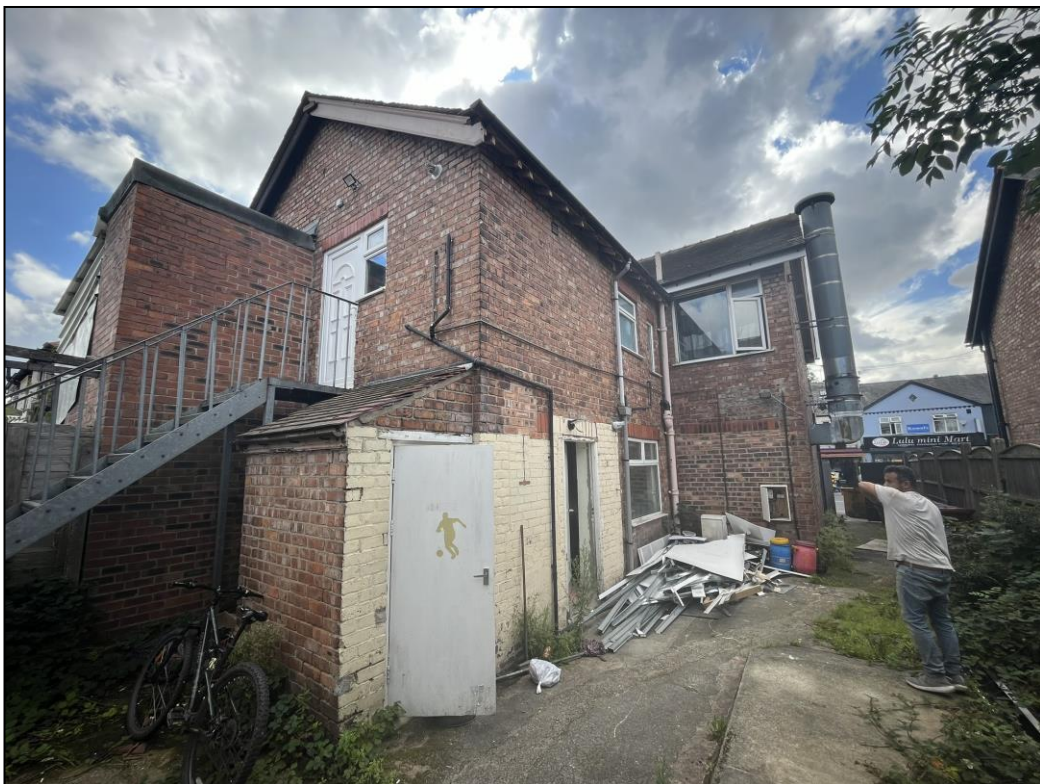
Figure 2. Rear of property
