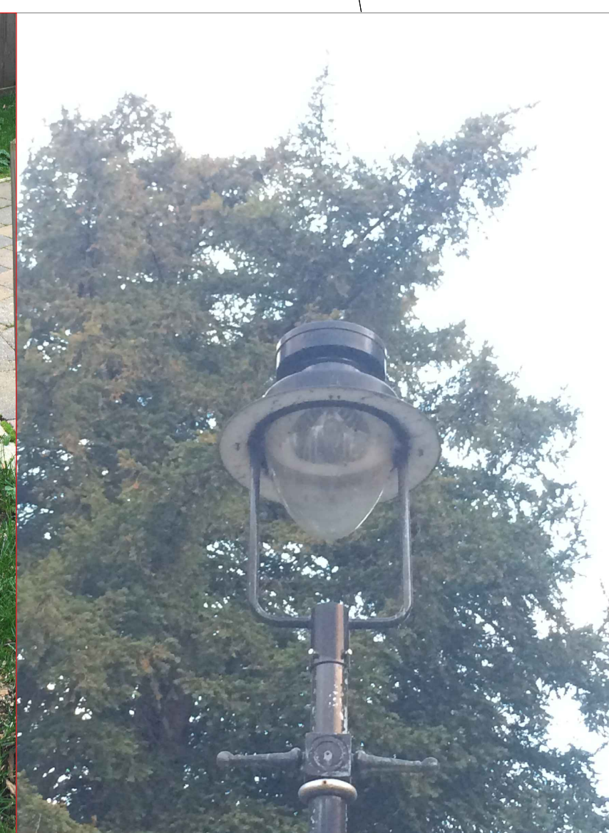
Existing Lights to be refurbished
