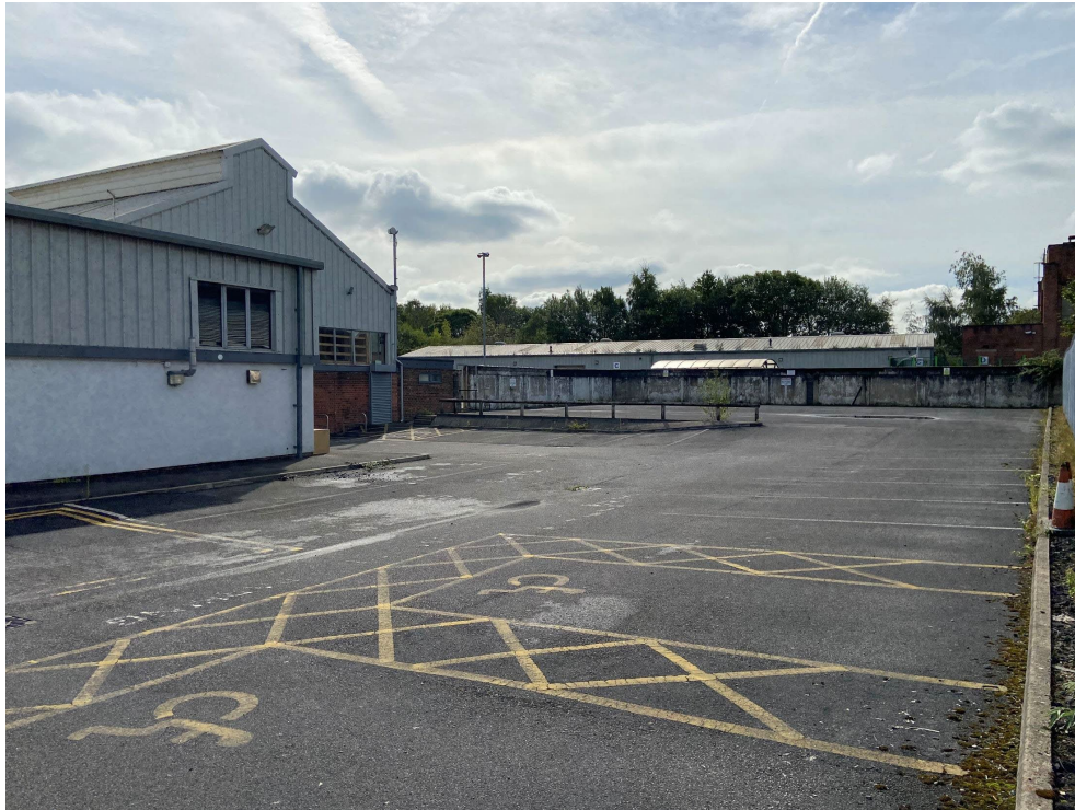
Figure 2 – Site photo looking south over the existing car parking area
