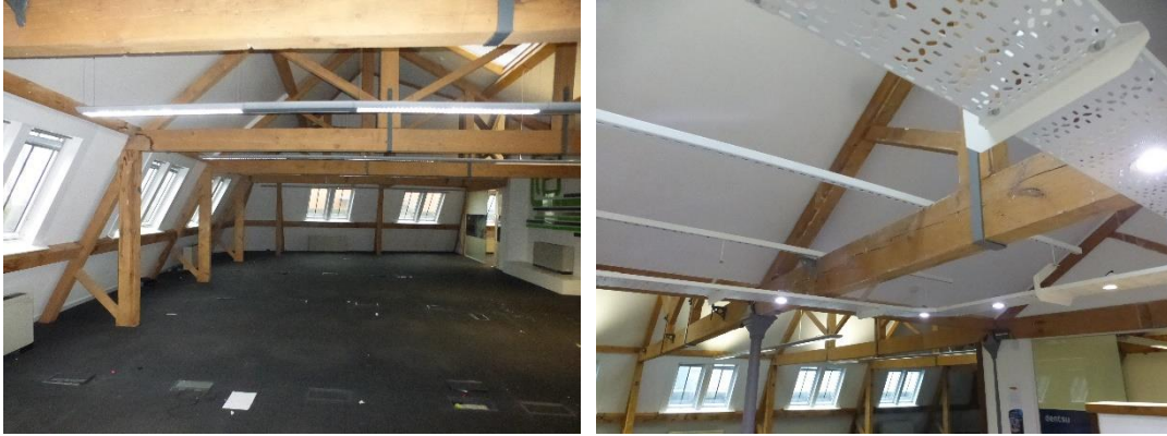
Typical 4 th Floor space
