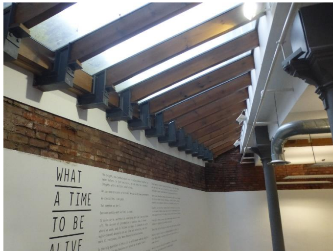
Glazed roof at rear elevation
