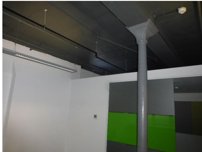
3 rd floor – Large beams to u/s 4 th floor encased in board.
