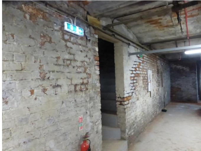
Entrance to former stair
