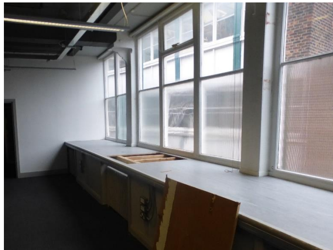
Glazed rear elevation. Note large cast iron bracket supporting timber floor beam
