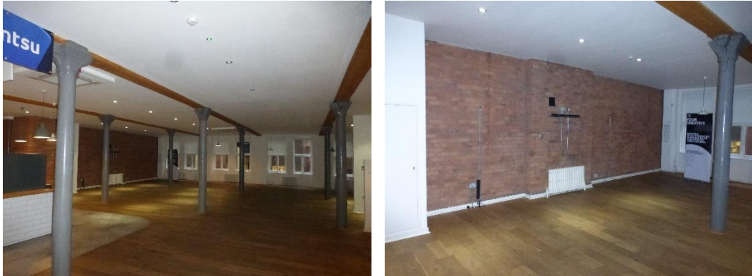
Typical ground floor arrangement with exposed brickwork to the main gable wall.
