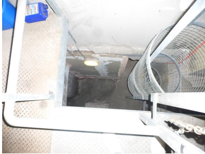
Ladder access to sub-basement.
