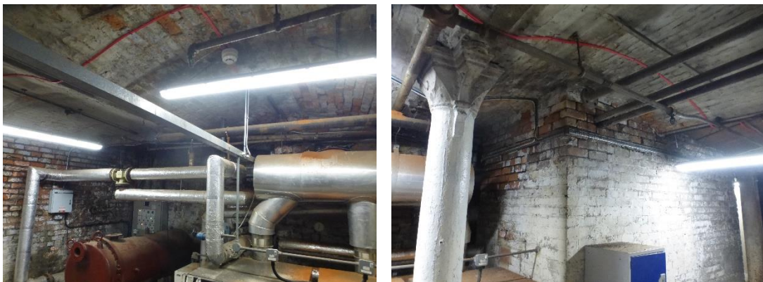
Brick arch / barrel vaulted soffit supported on cast iron beams, columns and loadbearing brick walls.
