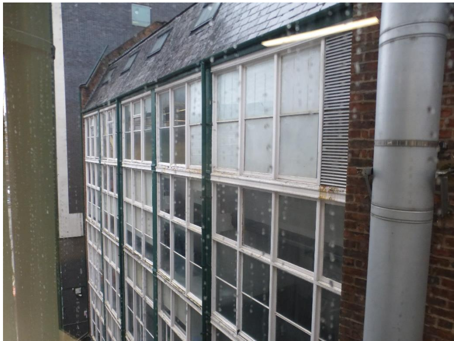
Main rear elevation viewed from 3 rd floor of 115 Portland Street
