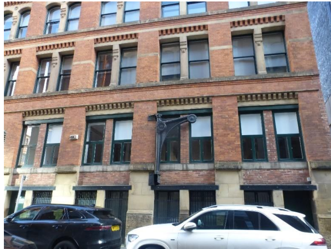
Lifting pulley to Dickinson Street elevation
