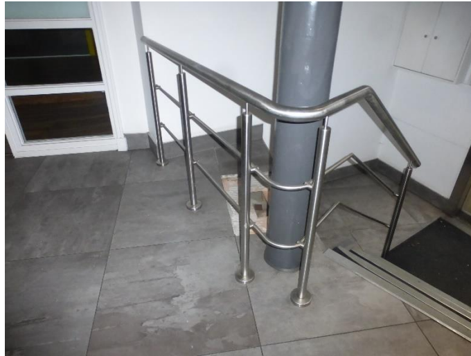
Stairs entrance off Portland Street.
