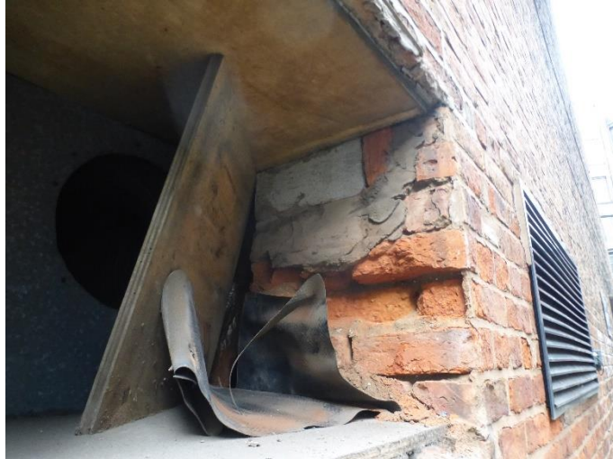
Opening in gable wall with louvre cover removed.
