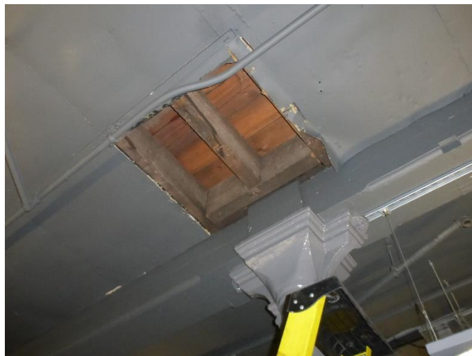
Typical floor joist arrangement at cast iron column heads with localised trimmer. Note feature column support heads to underside of main timber beams
