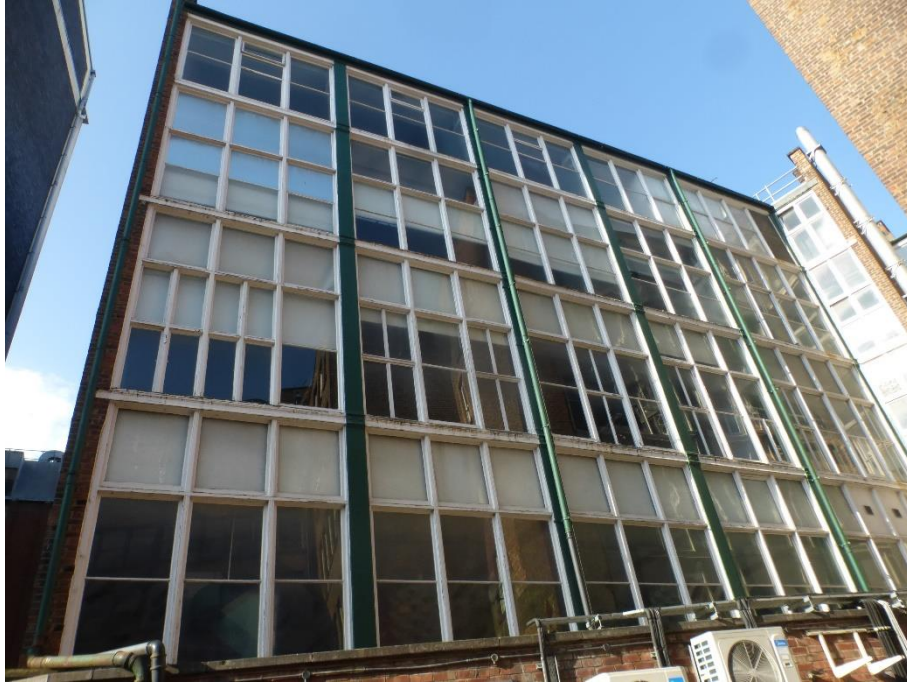
Main rear elevation viewed from car park
