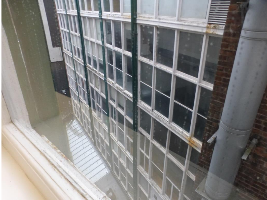
Main rear elevation viewed from 3 rd floor of 115 Portland Street. Small lean-to glazed roof above Lower Ground floor visible.
