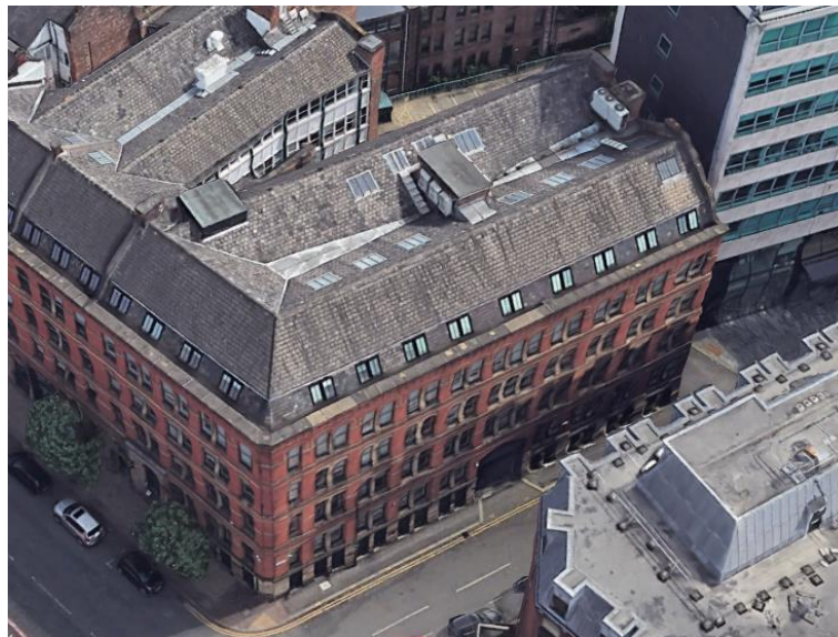
View from West
