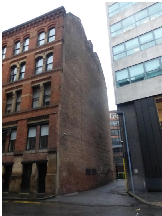
Gable elevation off Dickinson Street
