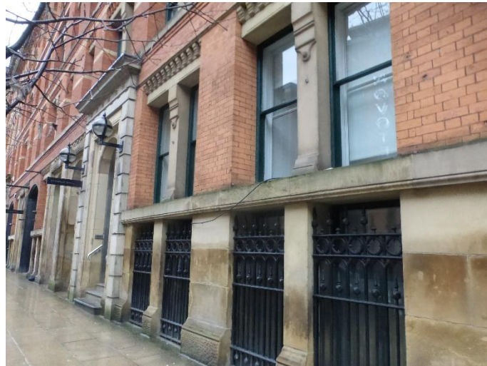
South corner looking towards the entrance door.
