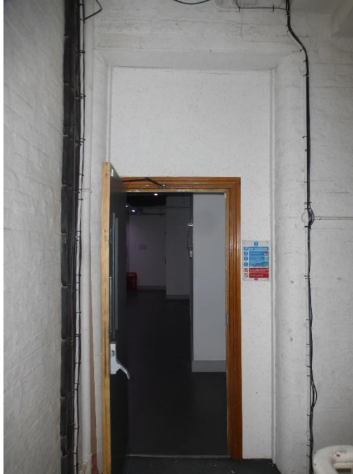
Door to fire escape stair (typical at most levels)
