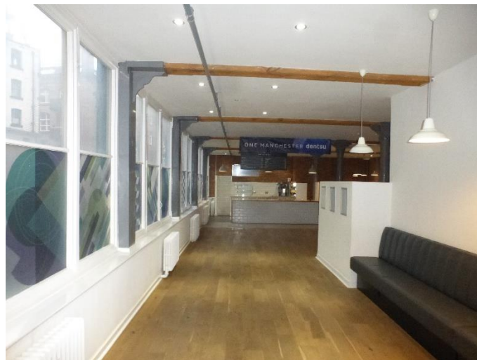
Cast iron brackets supporting floor beams off rear glazed elevation. Note the soffit is flat rather than sloping.
