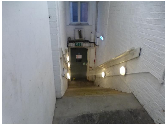
Fire escape down to Dickinson Street.
