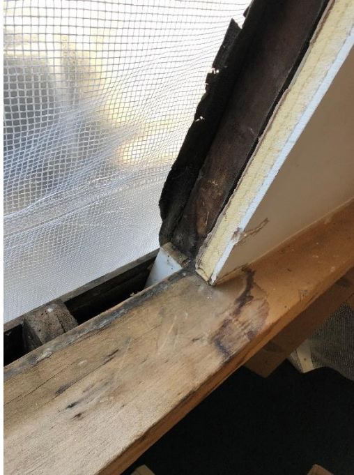
Record photo from 2019 showing the water staining to the purlins.
