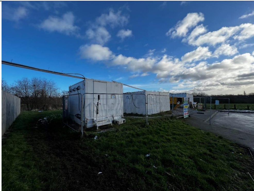
Figure 3: NM1 taken from the pavement (south-eastern facing)
