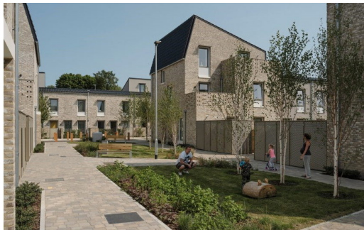
Example of an internal open space which comprises a pocket park environment with both defensible space to the rear gardens of the houses and shared amenity space and seating for the residents.
