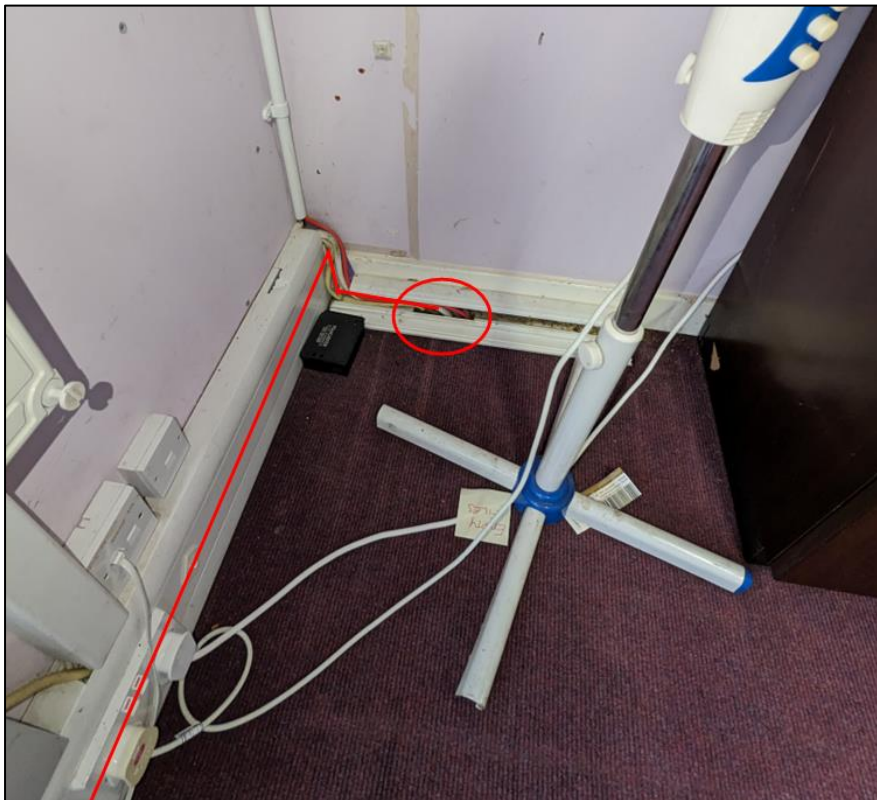
Appendix 5: The photograph above, taken in 024 Staff Room, indicates through the use of a red circle the point at which the aforementioned cable run enters 024 Staff Room. From this existing penetration the cable follows an existing cable run, terminating with the installation of AP3, the location of which is indicated by a green circle.
