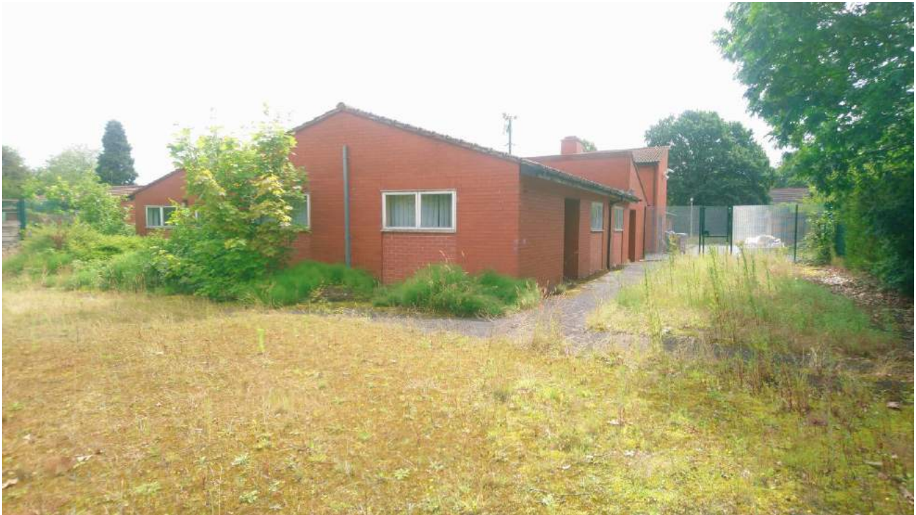
Photograph 5 View east towards the western elevation of the existing structure.
