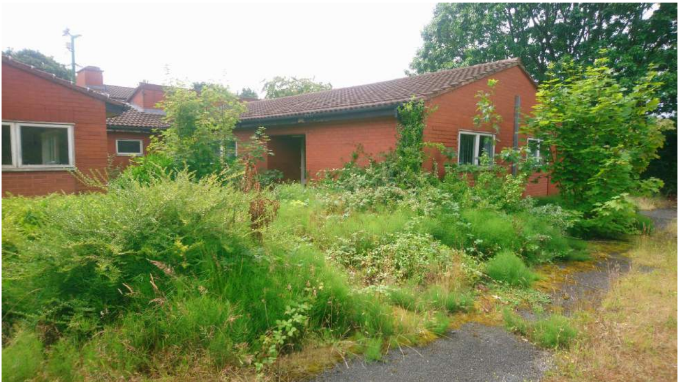
Photograph 6 View south-east towards the western elevation of the existing structure.
