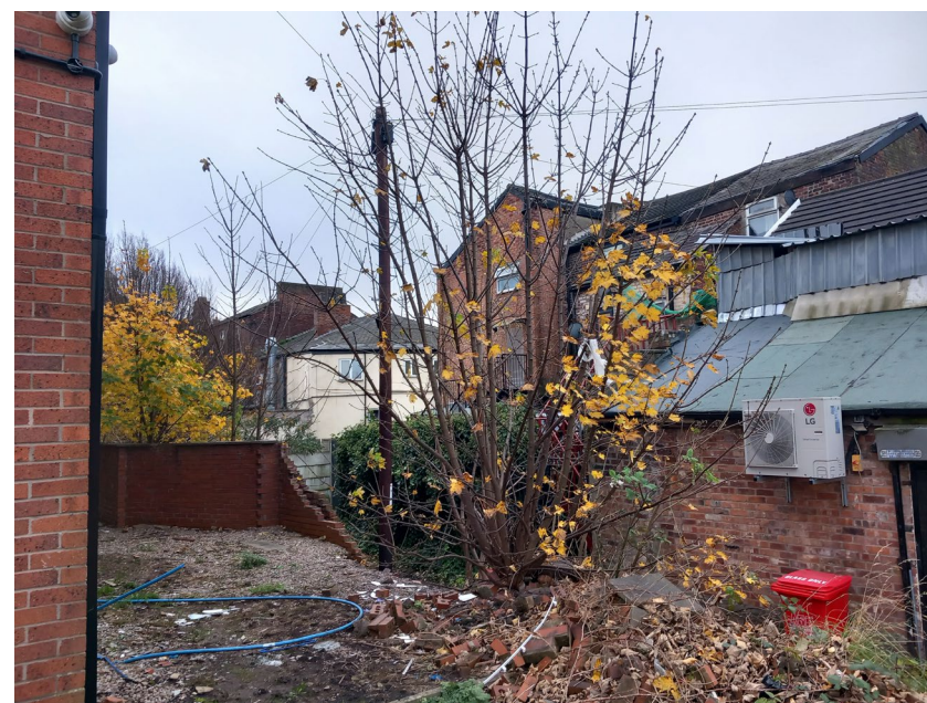
View to the rear of the existing block showing poor quality amenity space.
