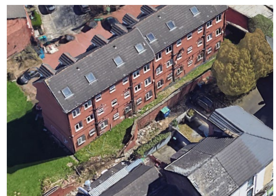
View to the rear of the existing block showing poor quality amenity space.
