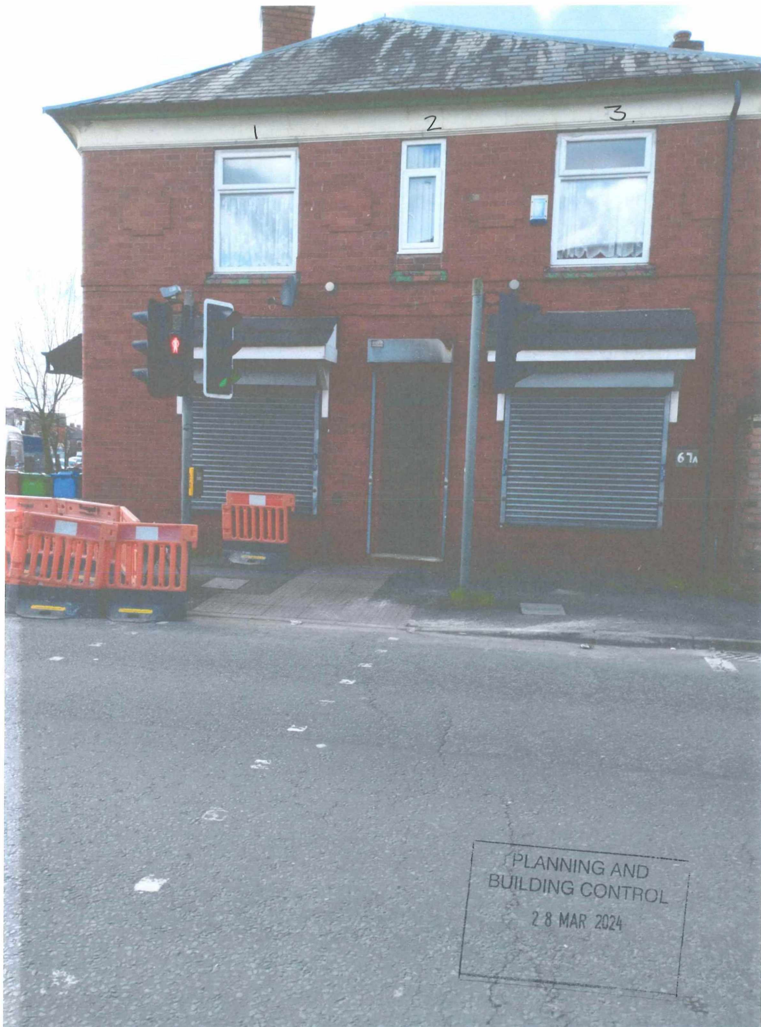
FRONT VIEW OF PROPERTY: Window 1 is the living room of 67A. window 2 is the kitchen of 67A. window 3 is the bedroom of 67A.
