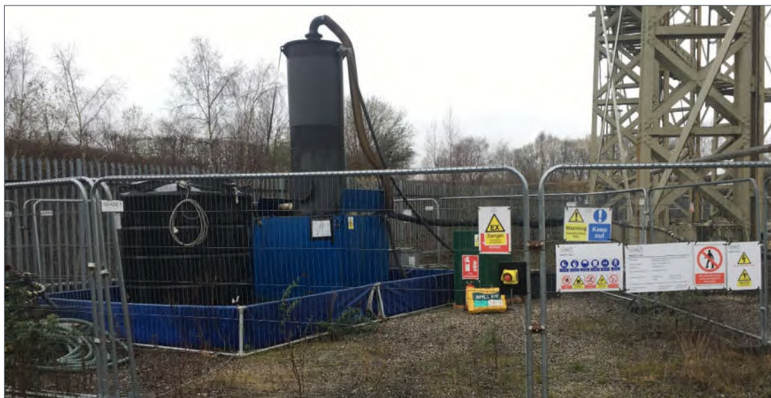
Figure 1 - Water Treatment Plant
