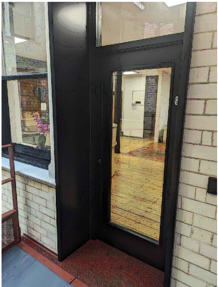
Photo 05 Existing entrance door to RSK area.
