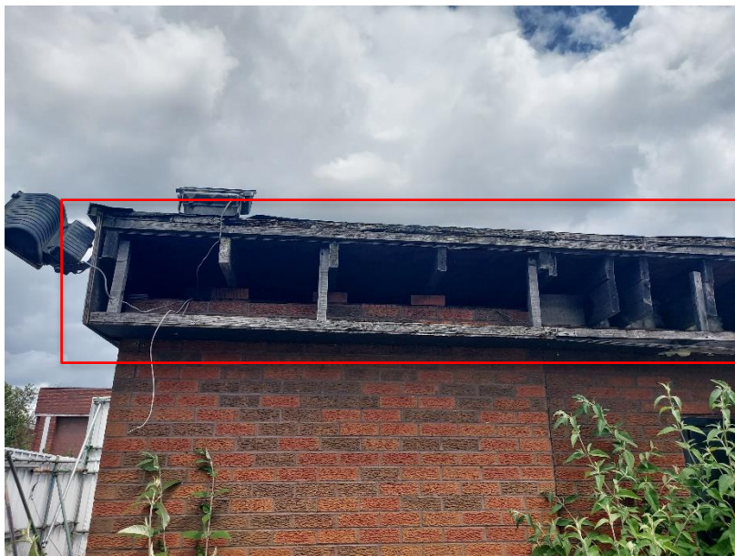
PLATE 2 SHOWING CLOSE UP OF ENTRY-WAYS INTO MAIN BUILDING
