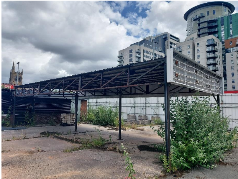
PLATE 3 SHOWING FLAT ROOFED EXTENSION
