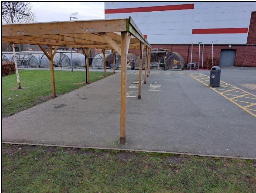
Photograph 1 showing the hardstanding bare ground at the science block location.
