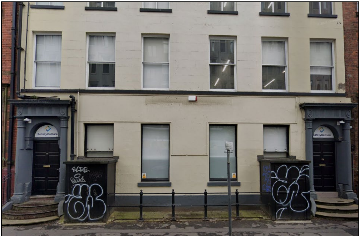
April 2021 - Signage for Safety Culture is apparent on the fanlights above the entrance doors on either side of the building.
