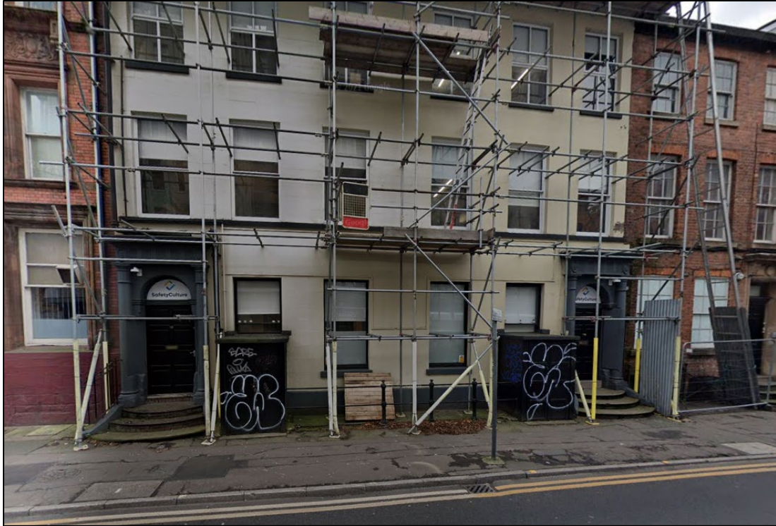
November 2020 – Signage for Safety Culture is apparent on the fanlights above the entrance doors on either side of the building.
