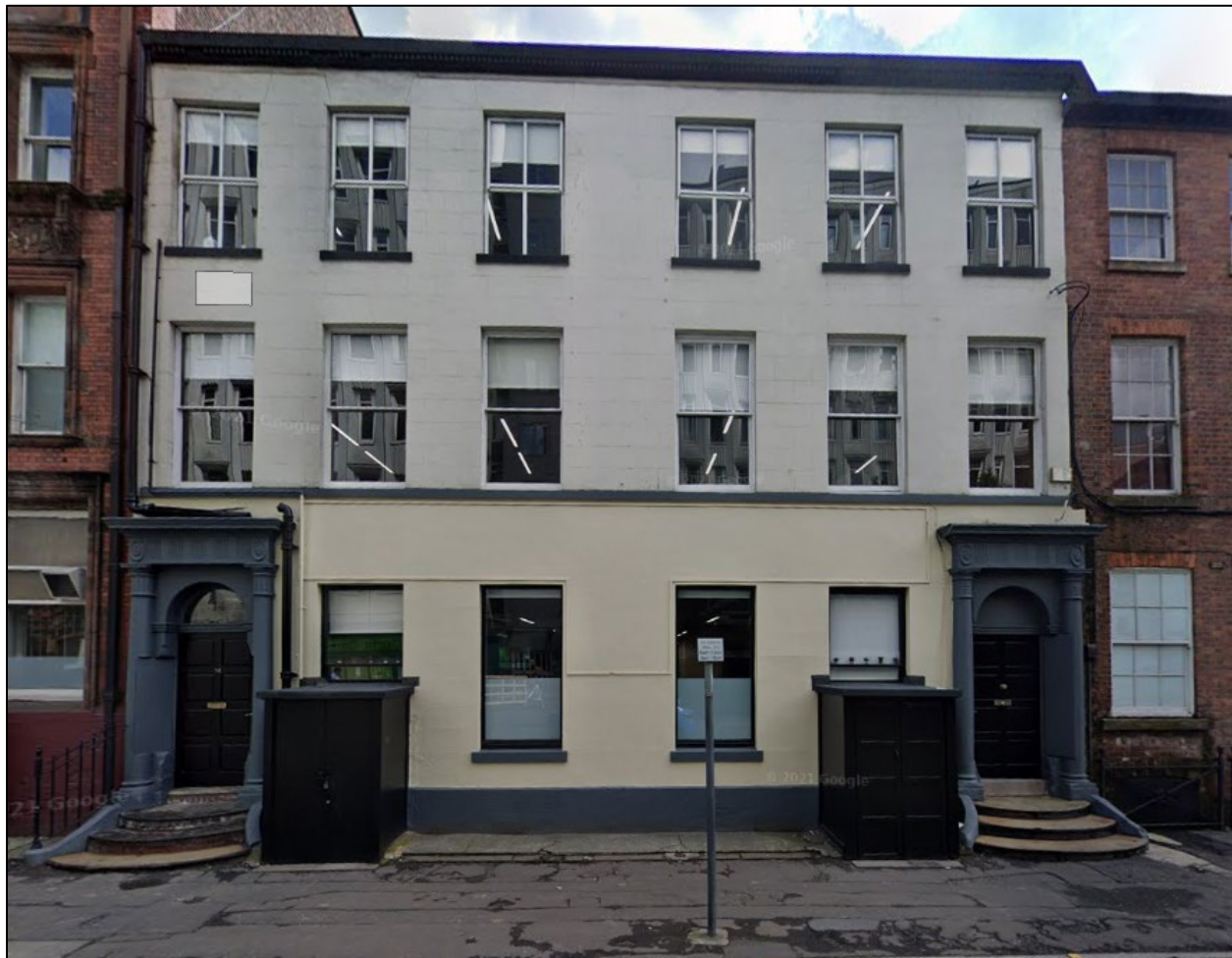
July 2019 - Following Extensive Refurbishment Works
