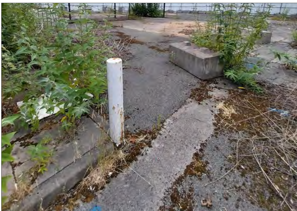
Plate 13 Photograph of the concrete surface within the Site, facing south-east
