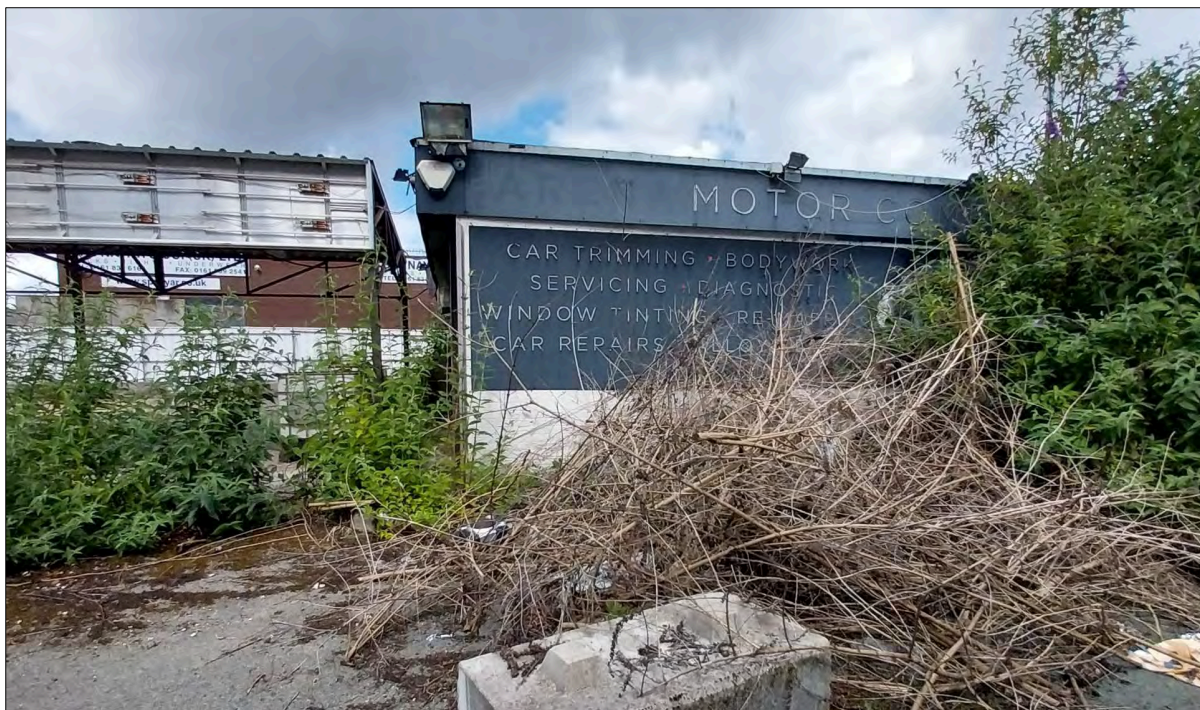
Plate 10 Photograph of disused garage within the Site, facing north-west
