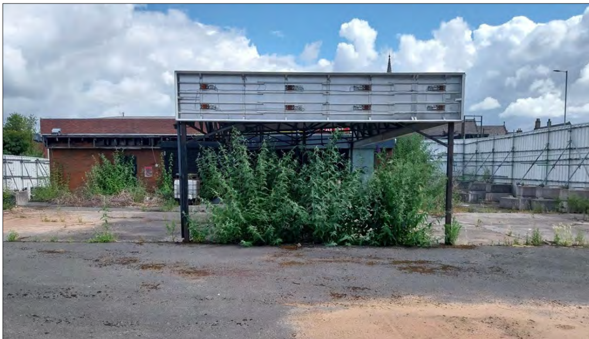
Plate 12 Photograph of the shelter within the Site, facing north
