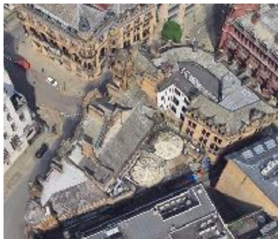
Fig. 2 Aerial view from rear of site
