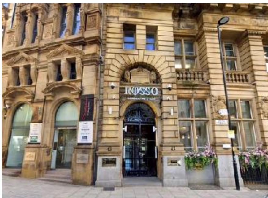
Fig. 5 Photo of former Rosso Restaurant entrance area
