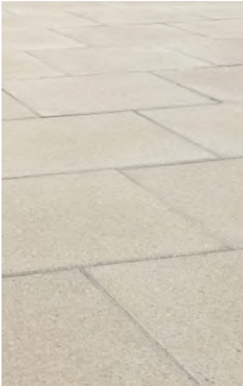
Street paving - concrete flags
