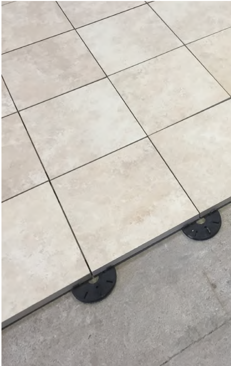
Roof terrace - porcelain tiles on pedestal and joist system
