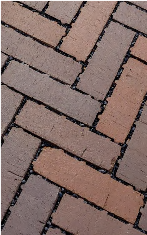
Podium paving - permeable setts
