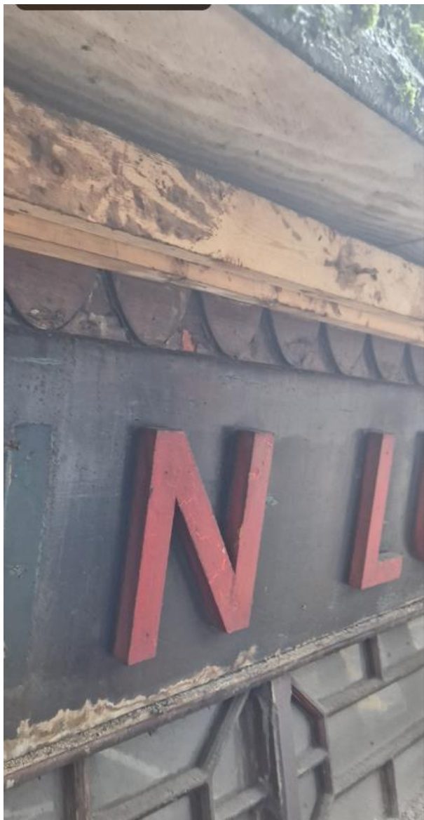
Photo 6: Detail of cornice feature.
