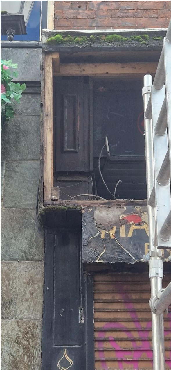
Photo 5: Detail of corbel feature.
