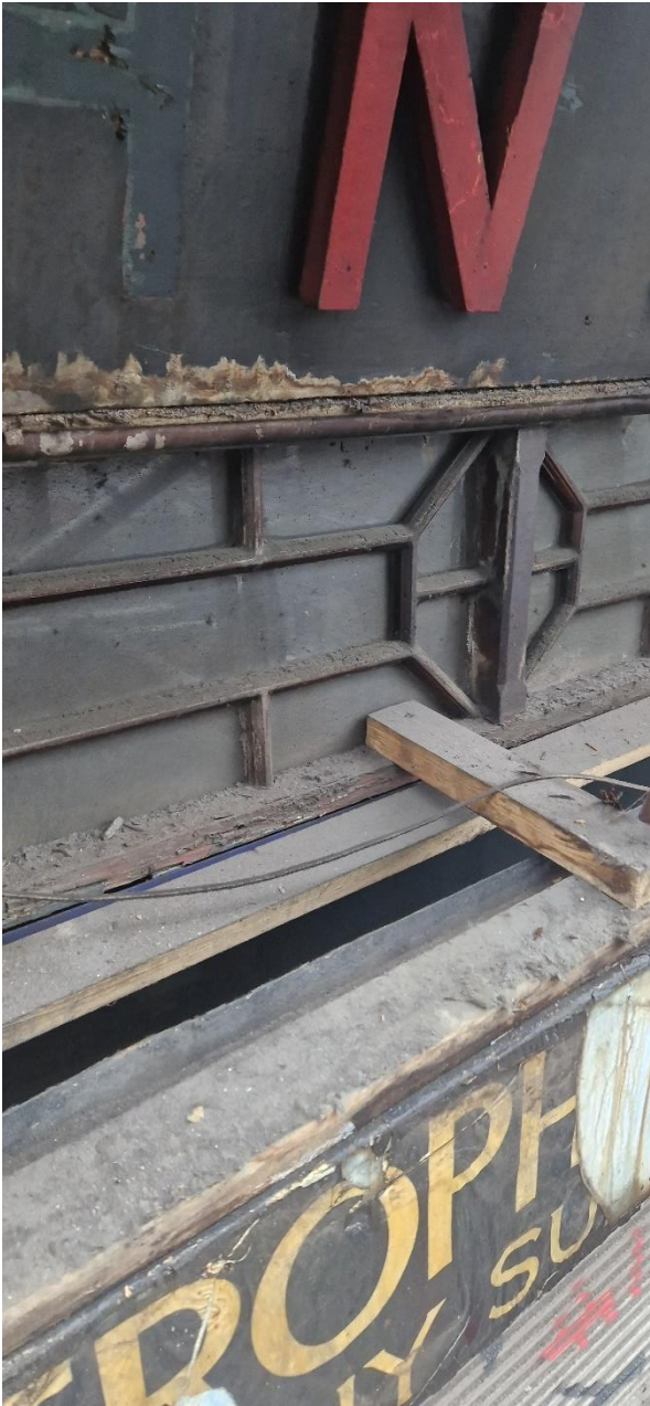
Photo 4: Detail of glazing above the main shopfront.
