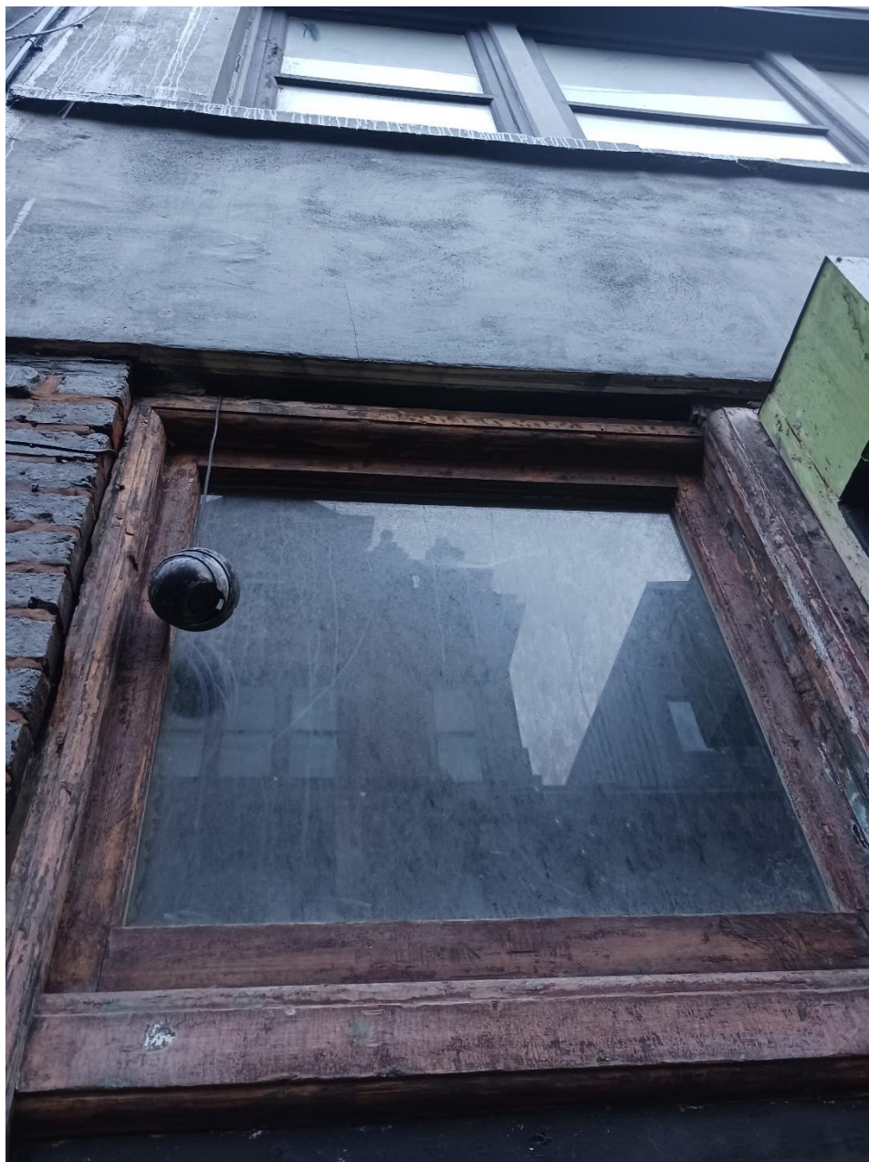
Photo 11: Detail of inserted timber shopfront.
