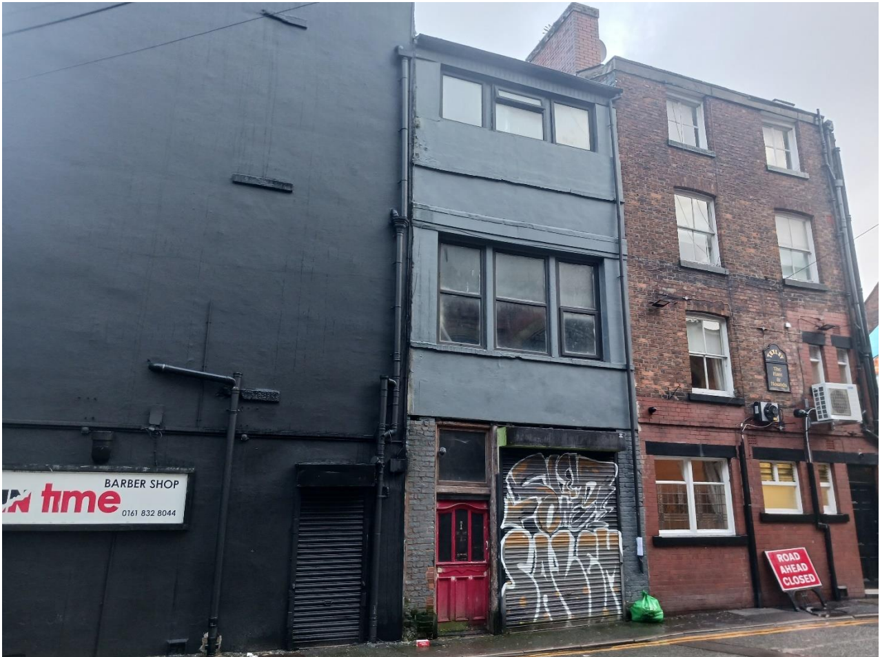
Photo 10: General shot of Salmon Street elevation.
