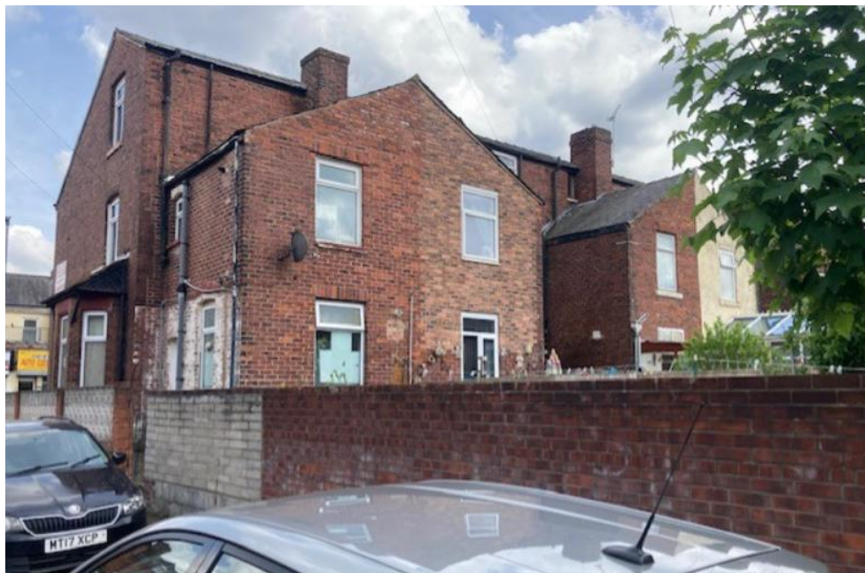
View of the application site rear
