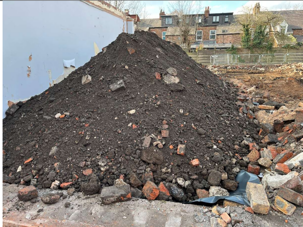
View of excavated contaminated material from around WS102 (referenced SP1).
