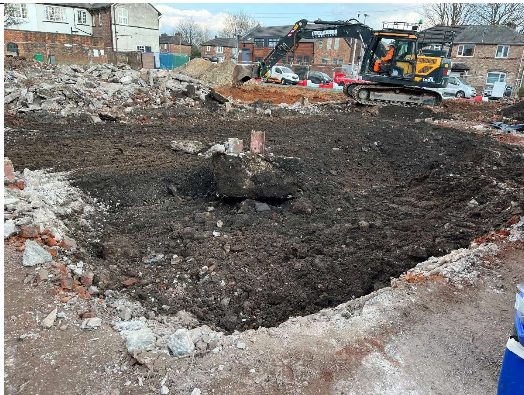
View of excavated delineation area around former WS102. All hydrocarbon contaminated material removed.
