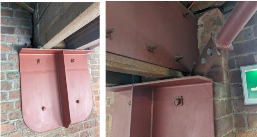
Figure 3-5 [left] 1980s strengthening plate detail at roof valley positions. [right] 1980s plate & diagonal brace, plus earlier strengthening plate detail to valley purlin
