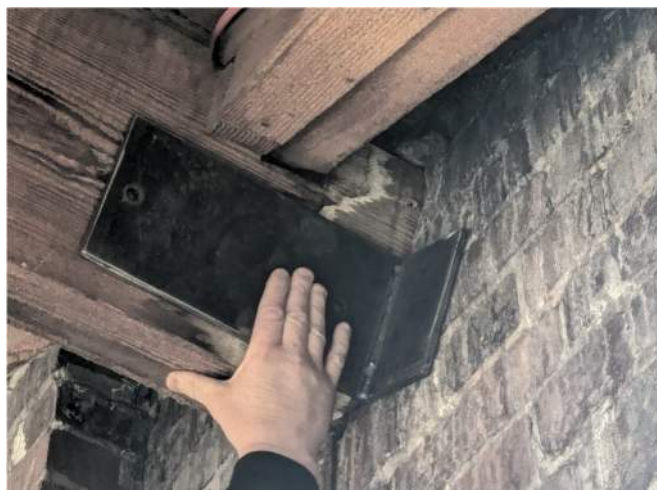
Figure 3-3 Site mock-up of standard bracket detail (unpainted)
