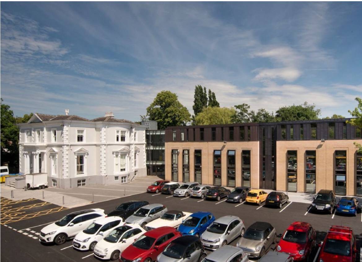
Ward Hall Building on Xaverian College Campus (Grade II Listed) & The Ward Hall extension.
