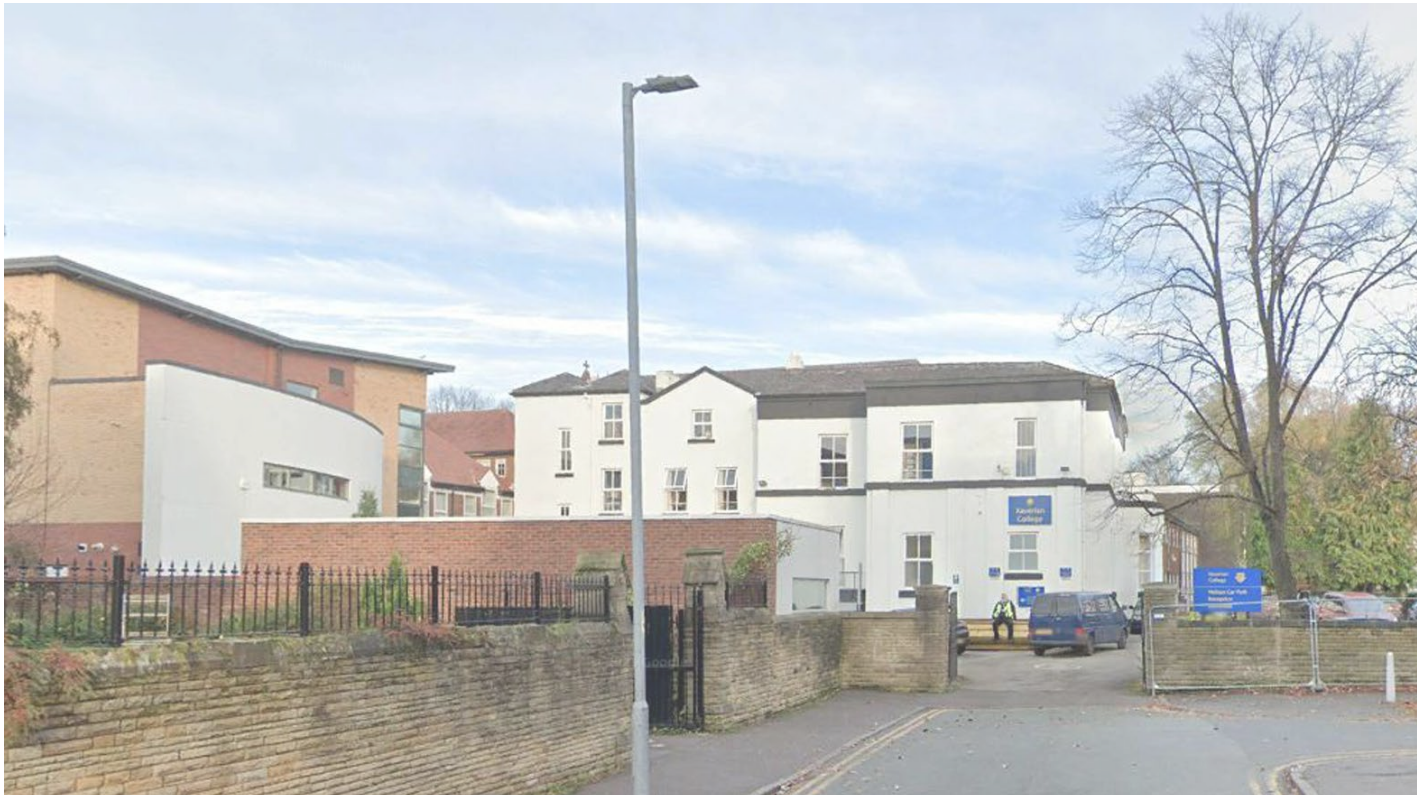
Existing site view looking East from Thurloe Street:
