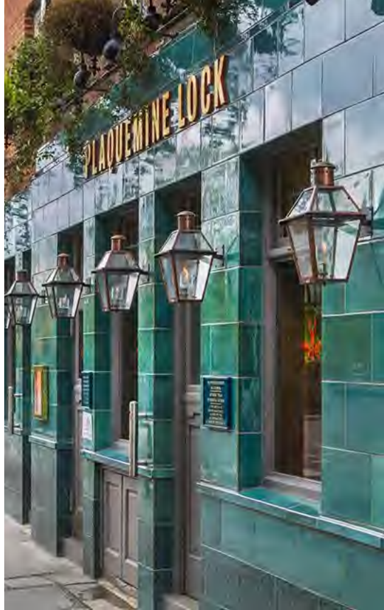
Fig. 141 Distinctive Faience Terracotta Base
