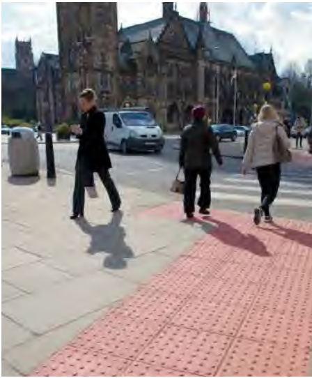
Fig. 191 Tactile Blister Paving Slab (to match existing in Great Ancoats Street)
