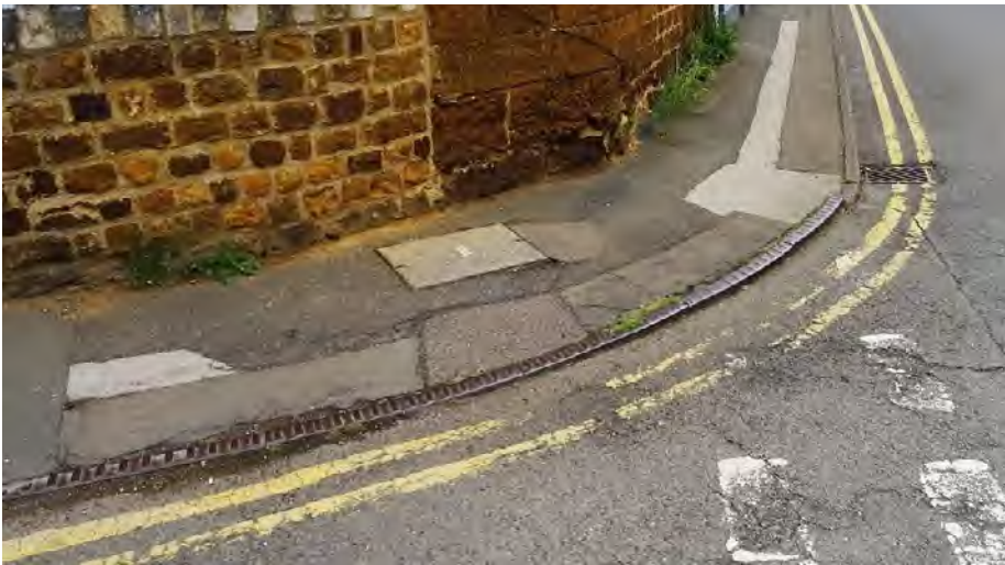
Fig. 195 Reclaimed steel kerb
