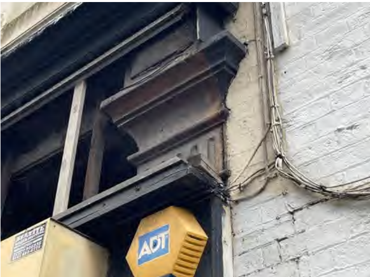
Fig. 70 Boarding covering stone details behind on 58 Lever Street
