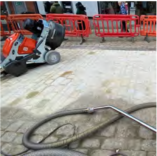
Fig. 194 Reclaimed cobbles ground with a vacuum assisted diamond grinder
