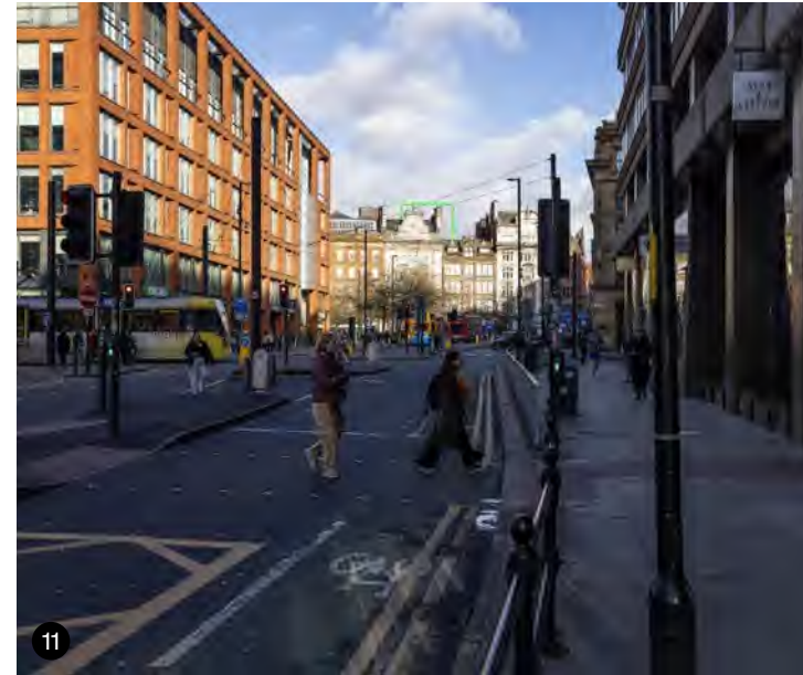
Fig. 125 View 11 - Verified View - Portland Street Northeast
