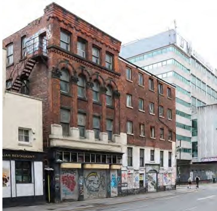
Fig. 34 No. 58 derelict Warehouse
