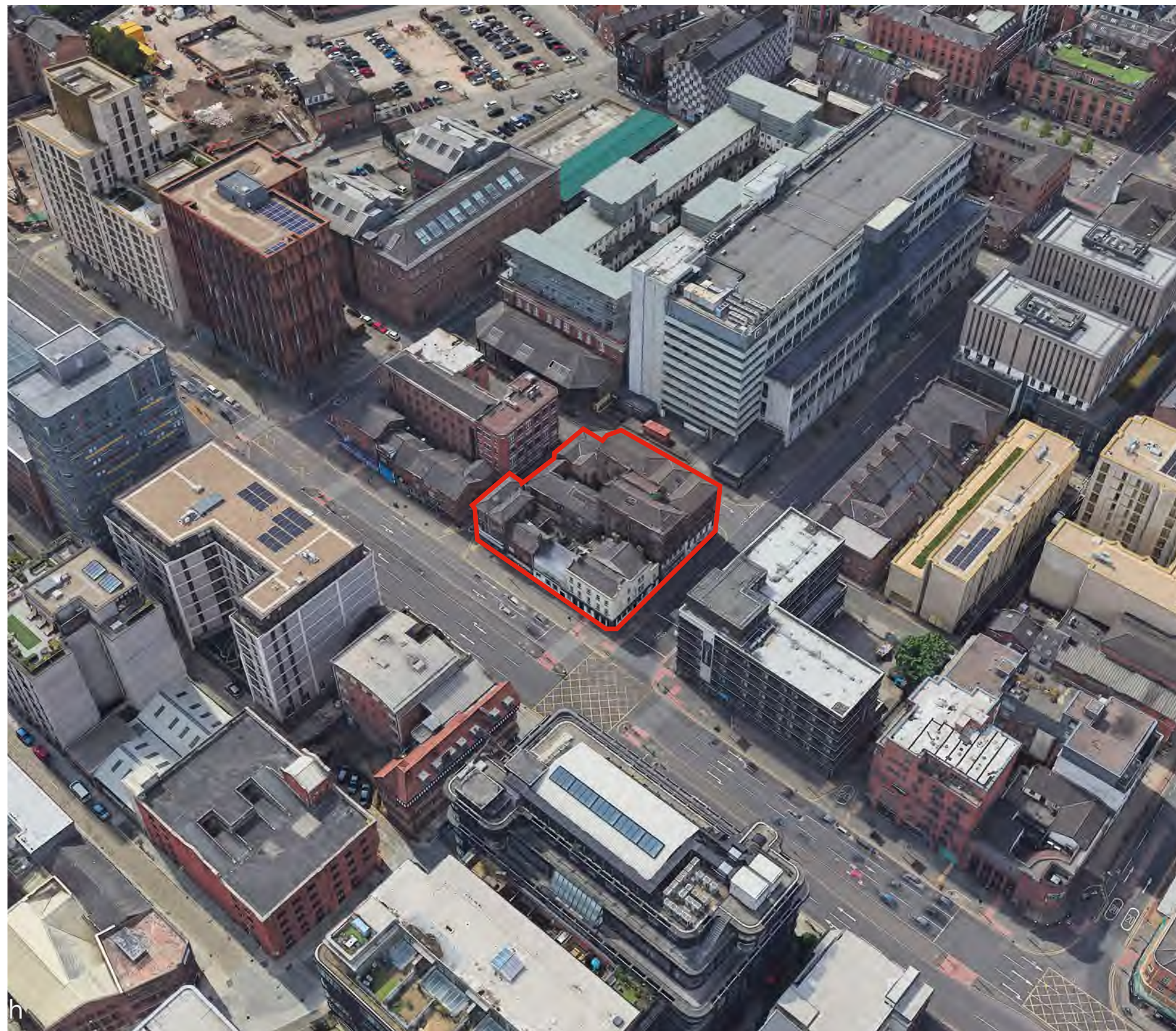
Fig. 46 Existing site aerial
