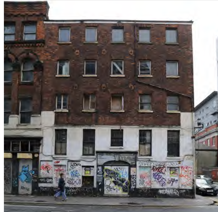
Fig. 35 No. 56 derelict Warehouse
