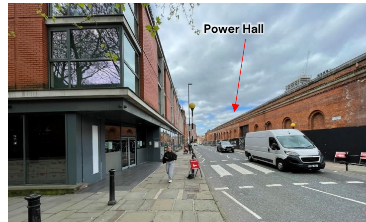
Plate 39: View west on Liverpool Road in front of the building.
