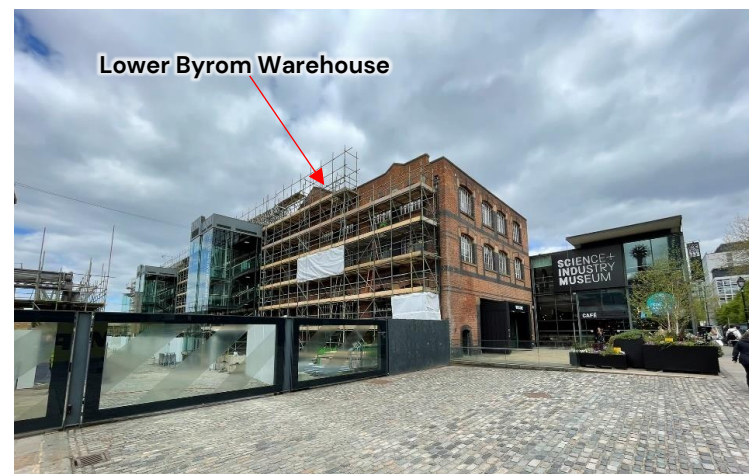
Plate 43: View north-east on Lower Byrom Street.
