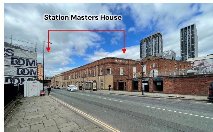
Plate 28: View of the building with the modern high-rise buildings to the rear.
