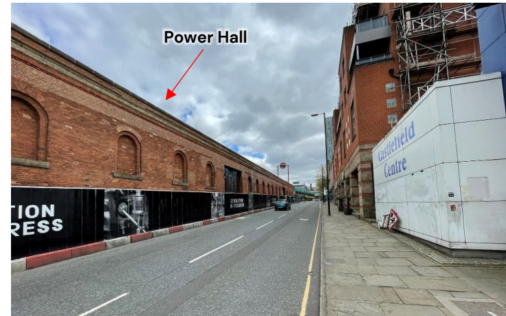
Plate 38: View east on Liverpool Road in front of the Power Hall.
