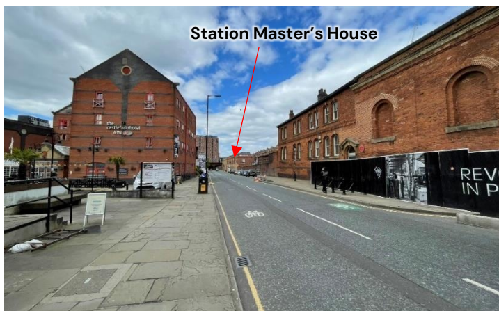
Plate 25: View of the Station Master's House from the east on Liverpool Road.
