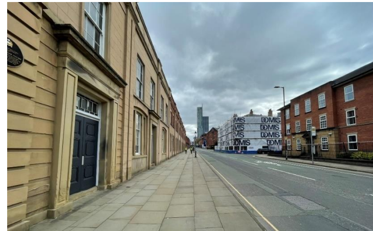
Plate 23: View east from the principal elevation of the Station Master's House.
