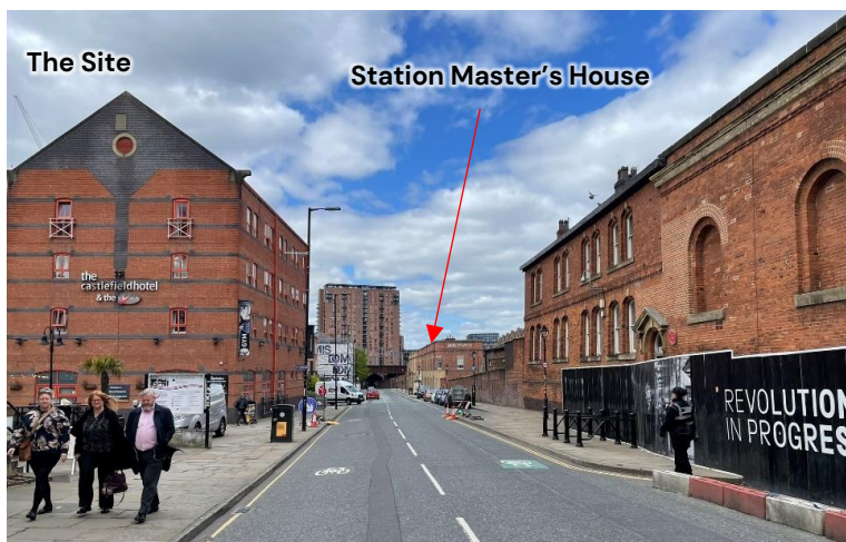
Plate 32: Co-views of the Site and Station Master's House.
