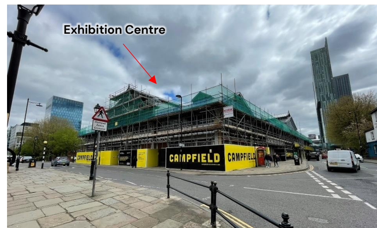
Plate 44: The Grade II Listed Exhibition Centre to the east of the former warehouse.
