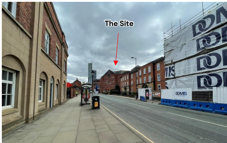
Plate 29: View towards the Site from the Station Master's House.
