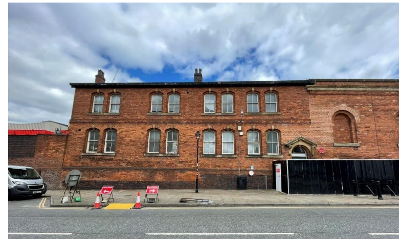
Plate 48: View of the Power Hall facing north from the Site.
