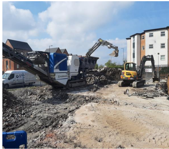
Image 11: Crushing works
