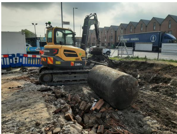
Image 11: Breaking out of interceptor
