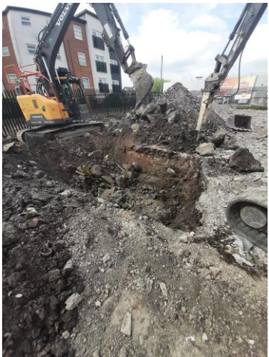
Image 12: Removal of interceptor
