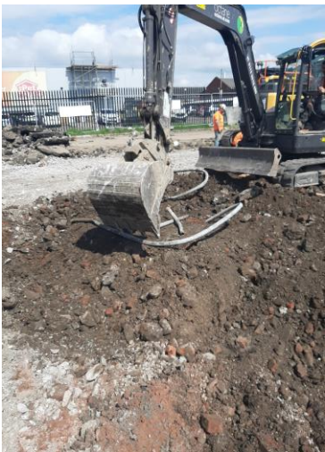
Image 12: Removal of interceptor
