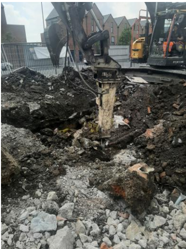
Image 11: Breaking out of interceptor
