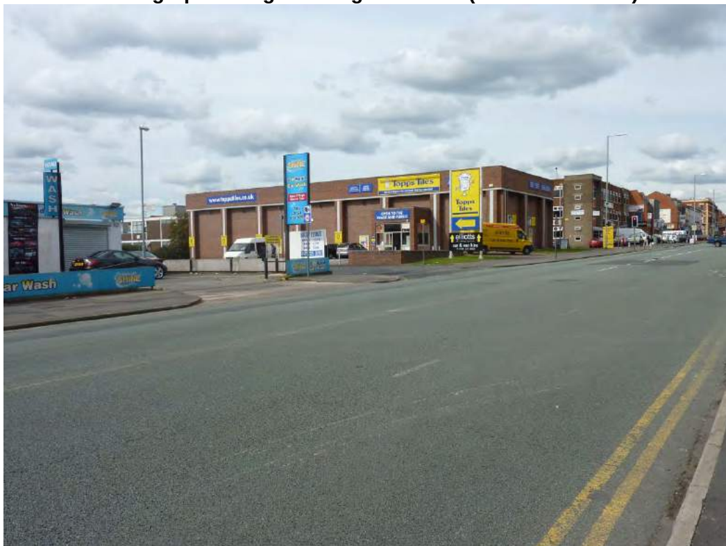
Photograph 4 Neighbouring land uses (north of the Site)
