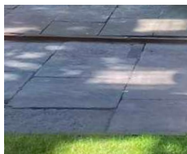
Existing sandstone reclaimed and re- purposed
