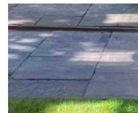
Existing sandstone reclaimed and re- purposed
