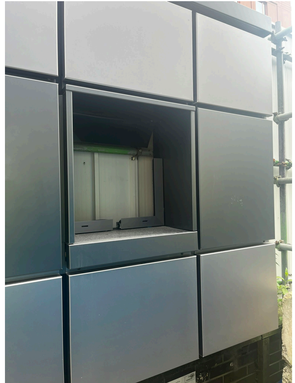
Cladding mock up arrangement with specified window (as agreed on site 02/04/2024)
