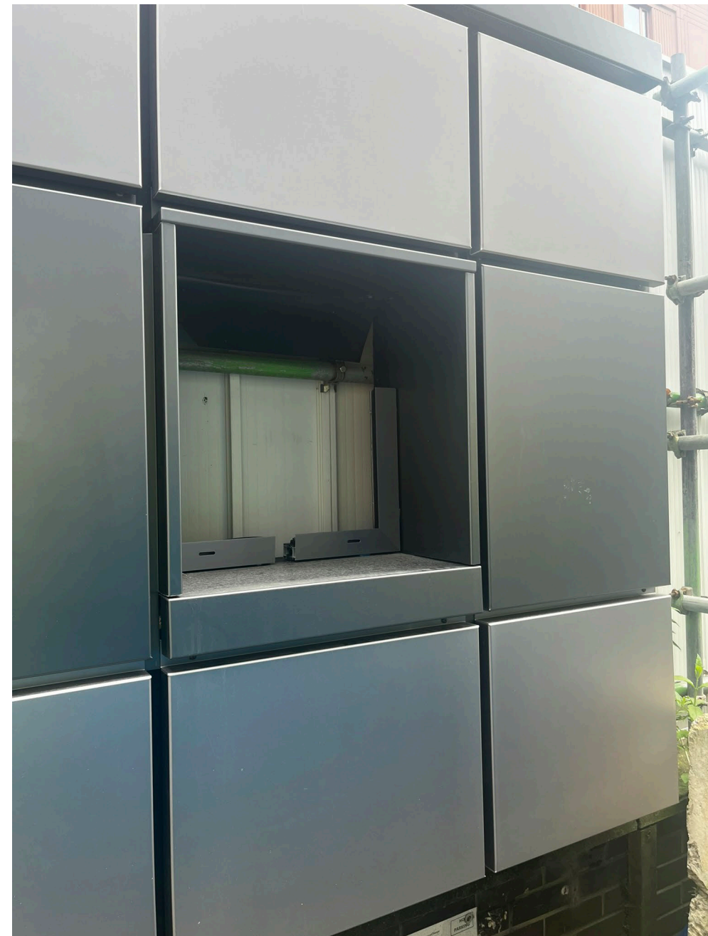
Cladding mock up arrangement (as agreed on site 02/04/2024)
