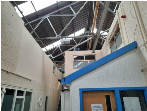
Plate 3: Building B1 Internal Area
