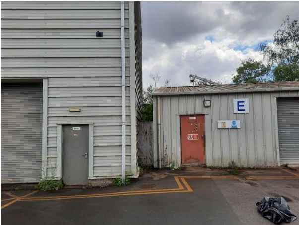
Plate 16: Building B6 Eastern Elevation (to left of photograph)
