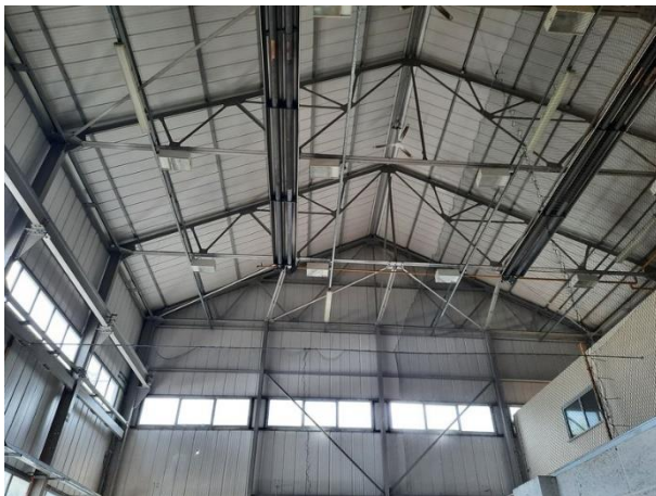
Plate 7: Building B2 Main Section Roof
