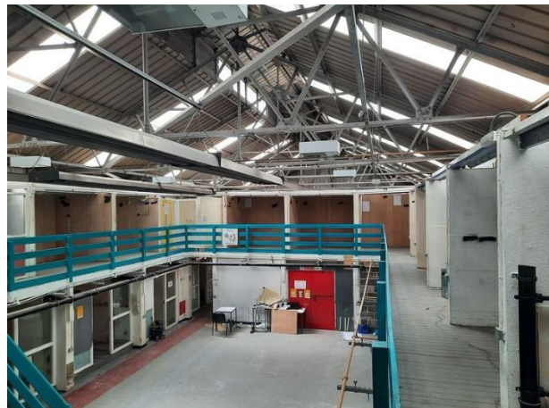
Plate 4: Building B1- Mezzanine Floor
