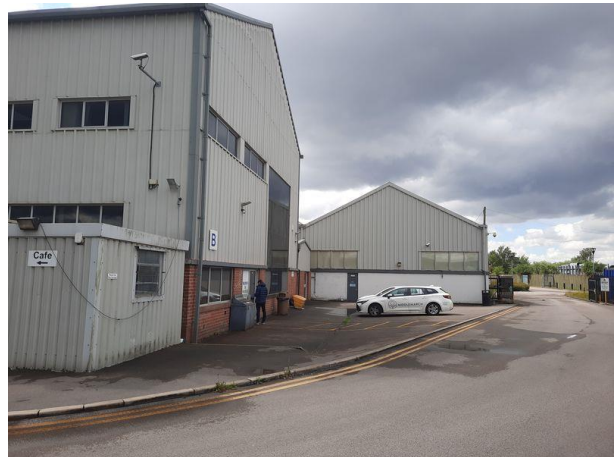
Plate 6: Building B2 Northern Elevation
