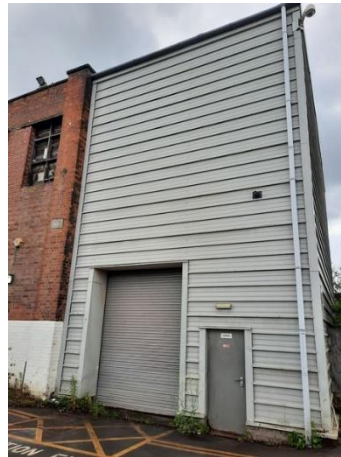
Plate 13: Building B5 Extension on Western Elevation
