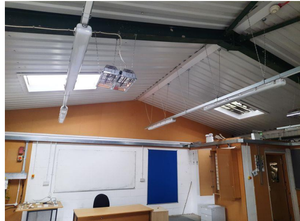
Plate 19: Building B7 Internal Area
