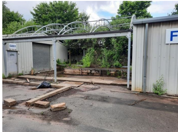
Plate 17: Buildings B7 and B8 Joined by Canopy Frame
