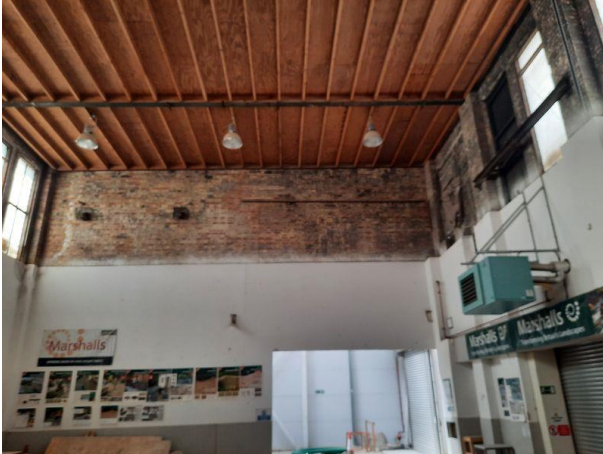
Plate 14: Building B5 Interior with Boarded Ceiling
