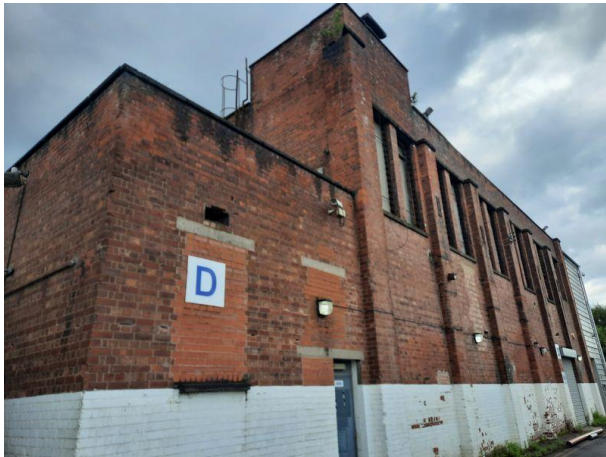
Plate 12: Building B5 Northern Elevation
