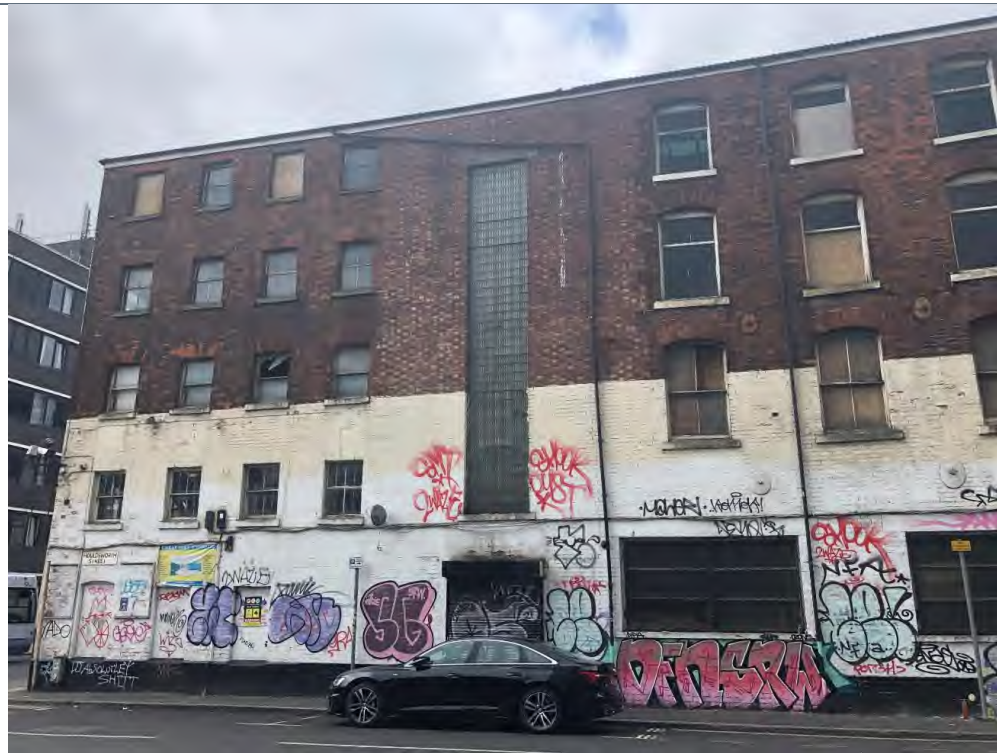
25 Houldsworth Street is four storeys in height, constructed from red brick and of four bays. The ground floor was altered in 1948 as part of the wider works by Drury and Gomersall to form two large window openings which sit in conflict with the upper floors. The first, second and third floors have an ordered arrangement of windows with slightly curved brick lintels and stone cills. A cast iron external fire escape stair has been added to the eastern bay.
