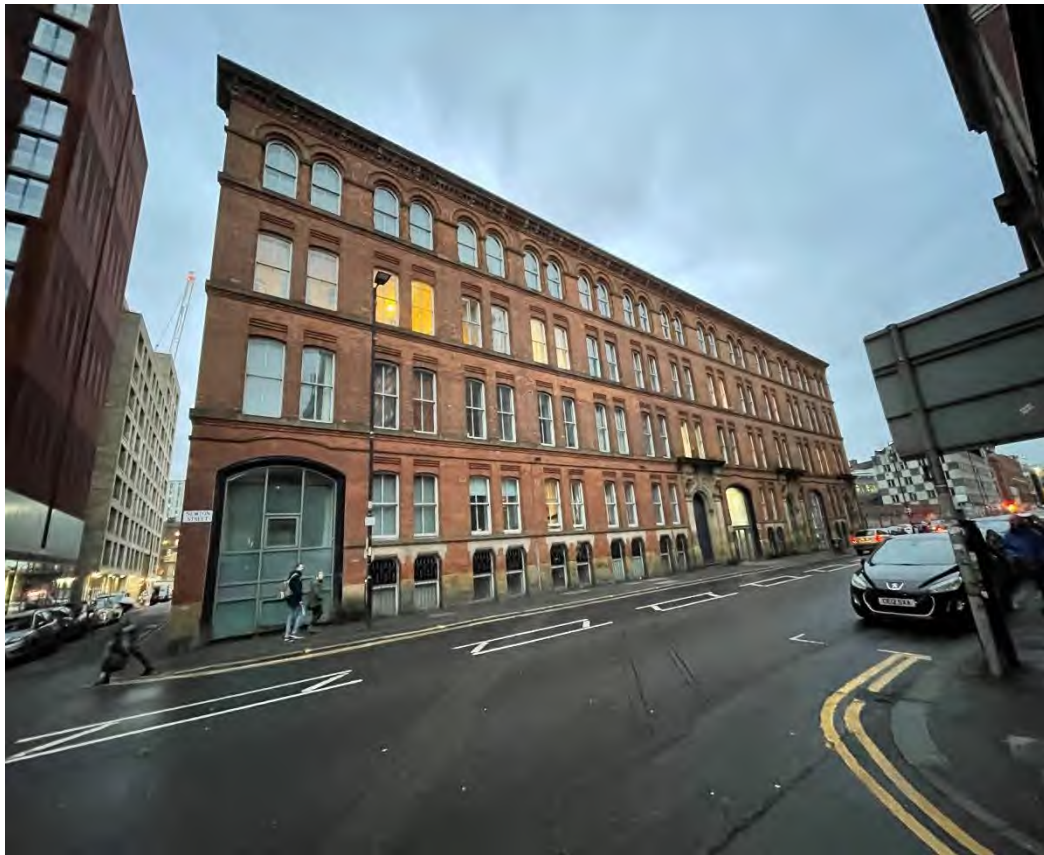
Figure 4.9: 72 to 76 Newton Street from Newton Street
