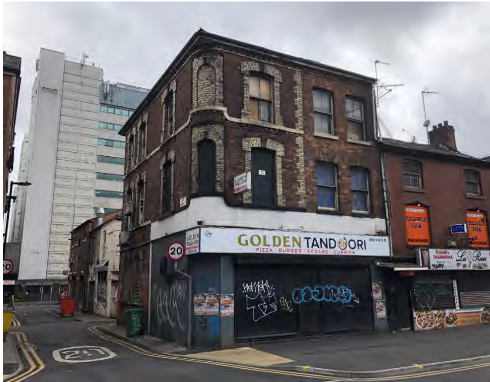
Existing Building: 40-42 Great Ancoats Street
