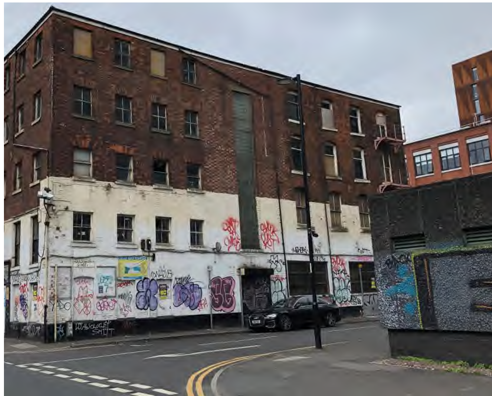
25 Houldsworth Street is four storeys in height, constructed from red brick and of four bays. The ground floor was altered in 1948 as part of the wider works by Drury and Gomersall to form two large window openings which sit in conflict with the upper floors. The first, second and third floors have an ordered arrangement of windows with slightly curved brick lintels and stone cills. A cast iron external fire escape stair has been added to the eastern bay.
