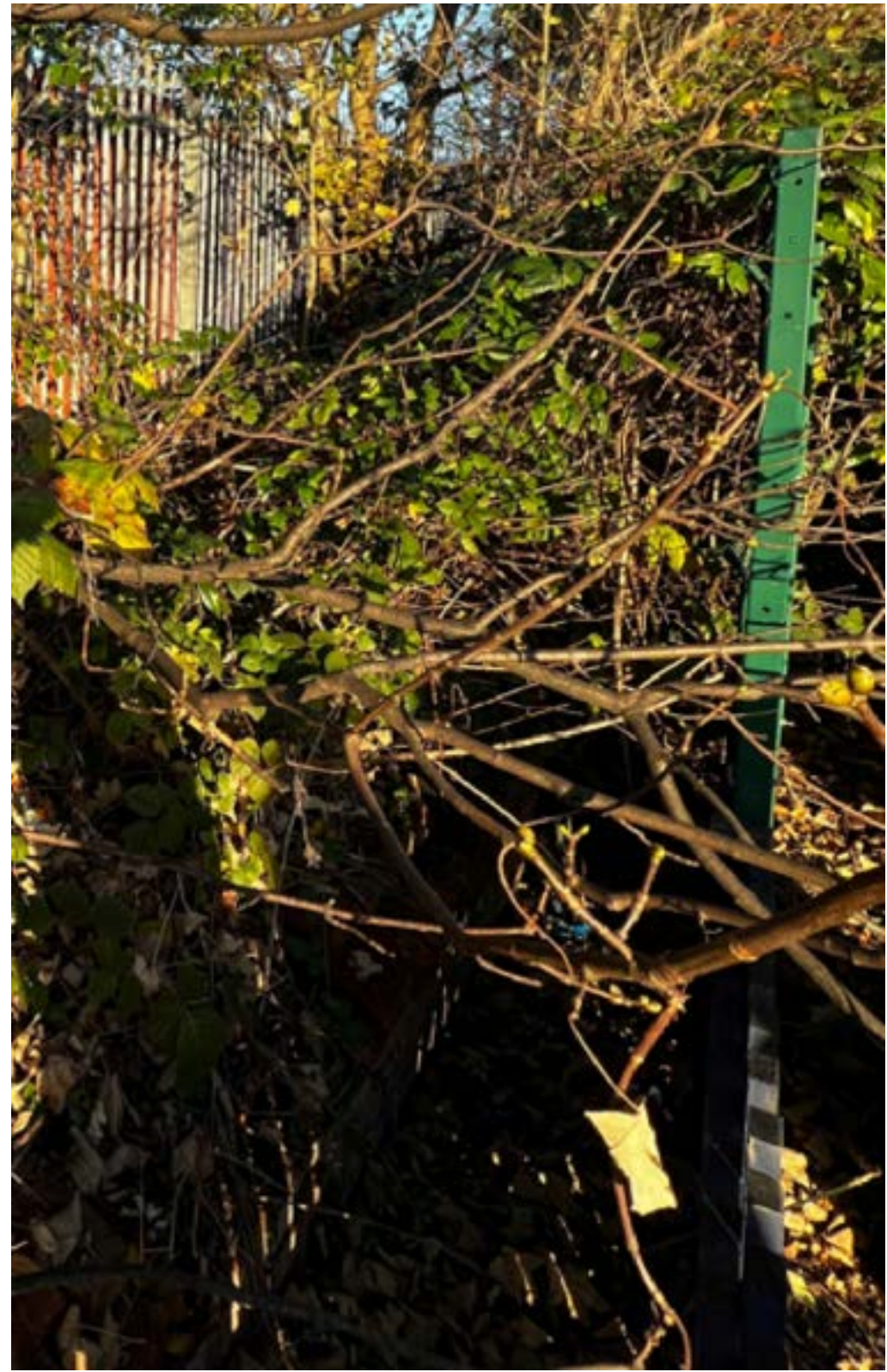
EXISTING RIGHT OF WAY - OVERGROWN
