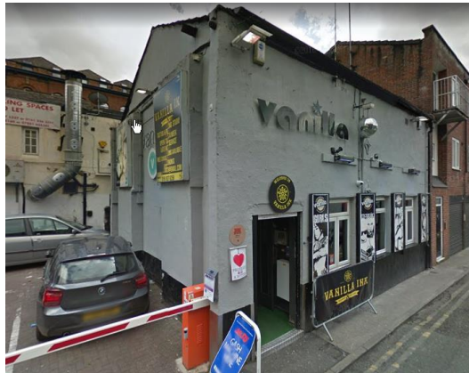
Figure 1 Street view of site
