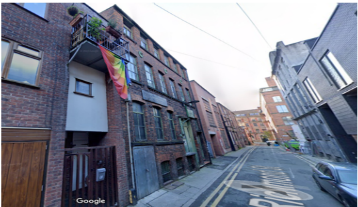
Fig. 8: The warehouse at 51-53 Richmond Street
